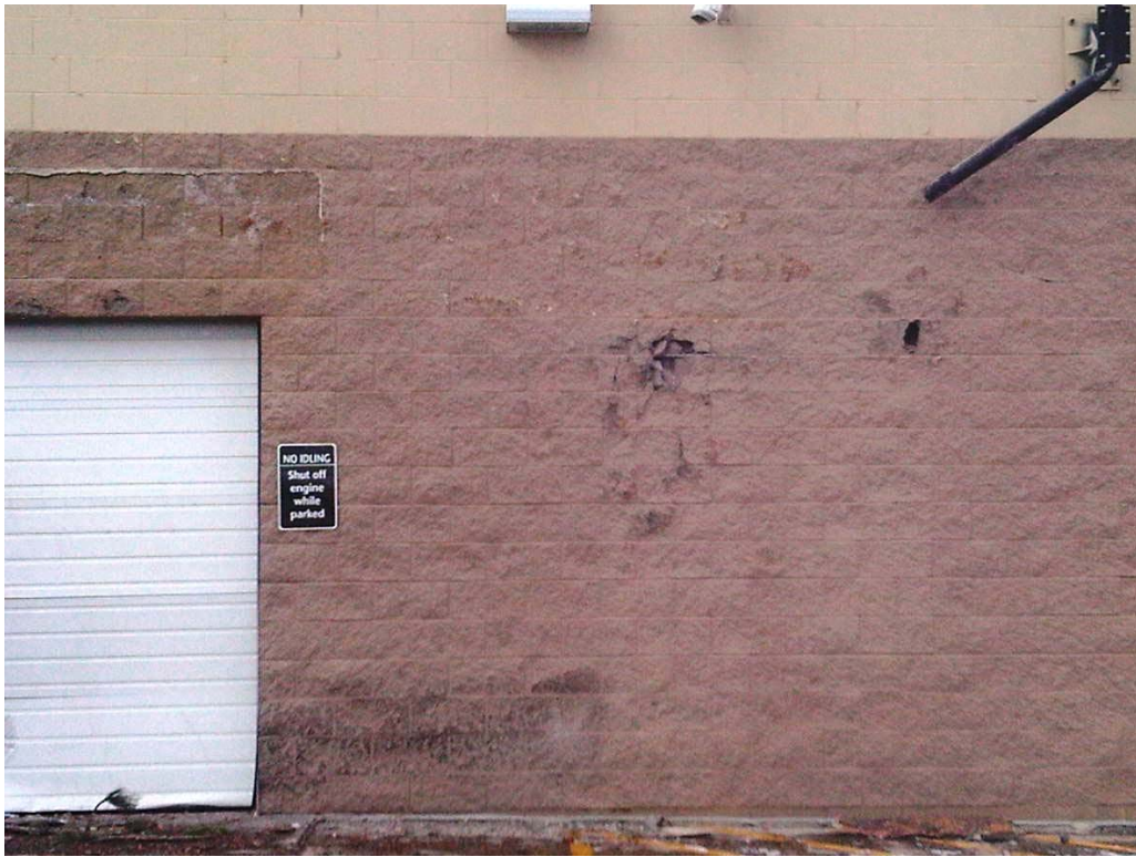
Figure 6 Wall Damaged by Impact
