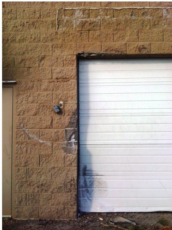
Figure 7 Wall and Steel Door Damaged by Impact
