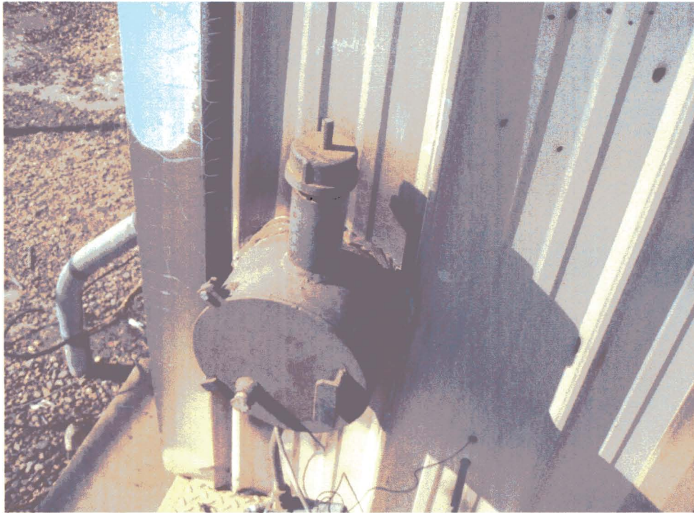
Figure 5. Building Heater Ignition Source Located Outside of Door
