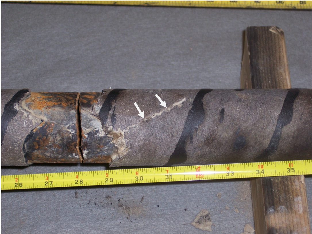
Figure 11. Disbonded area near crack where coating remained intact. The boundary of the disbonded area is characterized by a white deposit (denoted by arrows).
