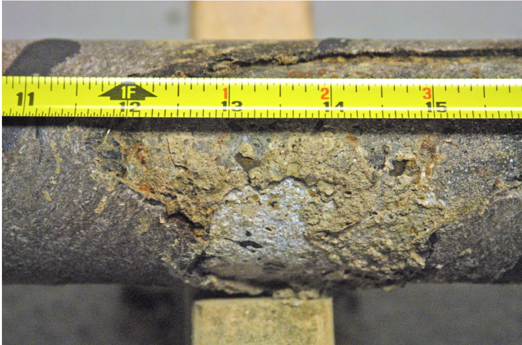
Figure 9. Disbonded area, side of pipe, located about 13 inches from End A
