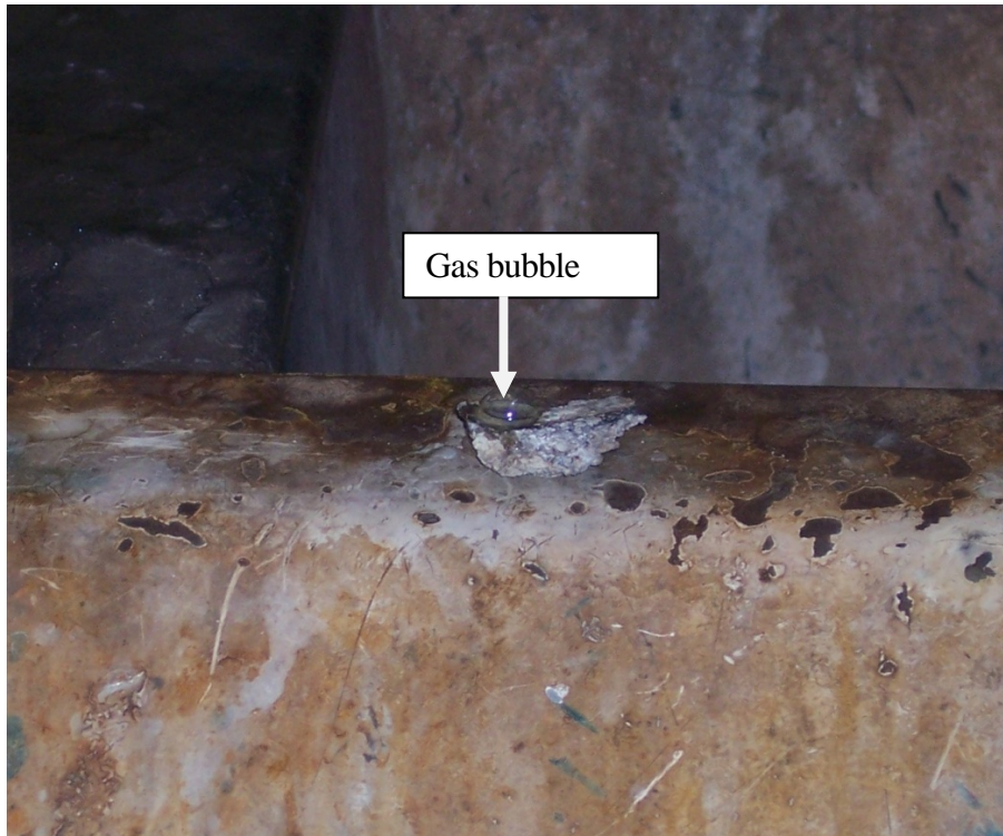
Figure 12. Effervescence of white deposit when treated with dilute HCl.
