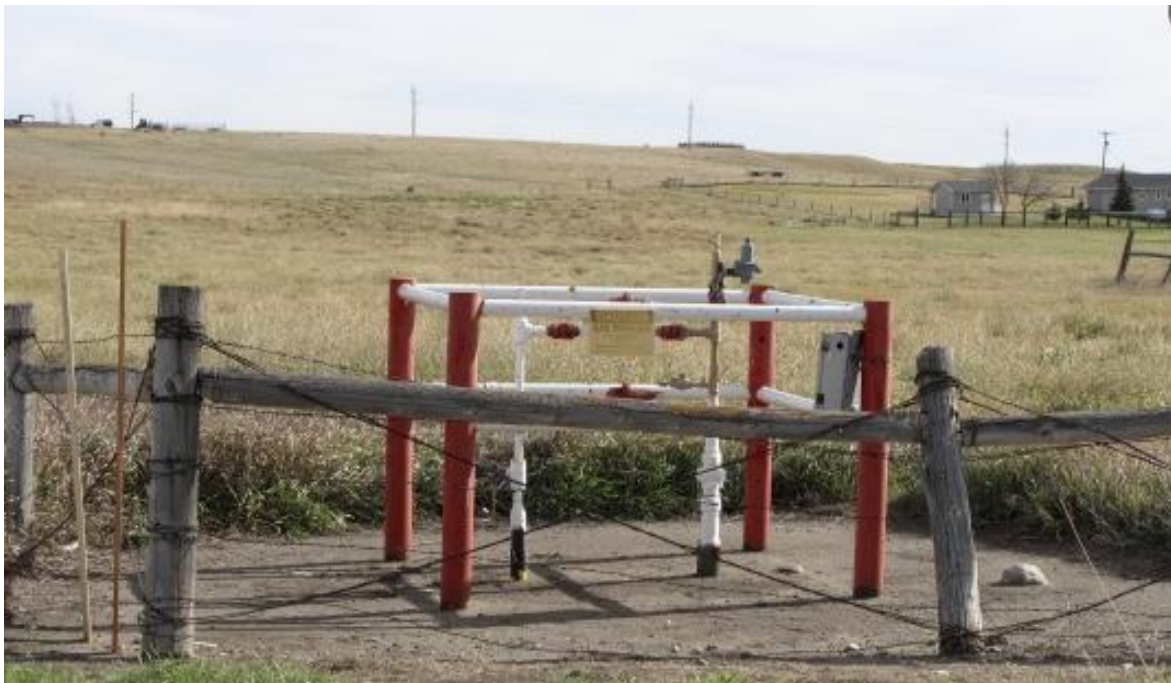
48.) Tap for City of Glenham off of 3" lateral.
