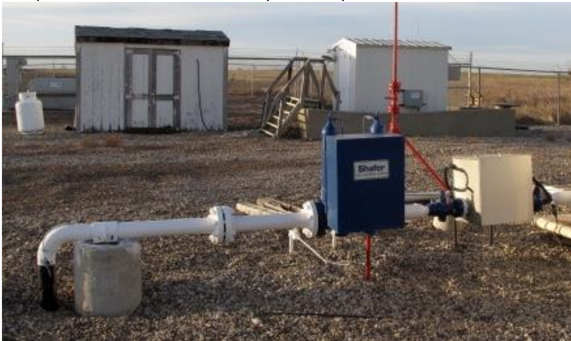
4.) Additional shut off valves pertinent to MINA Station for South Dakota Intrastate Pipeline.
