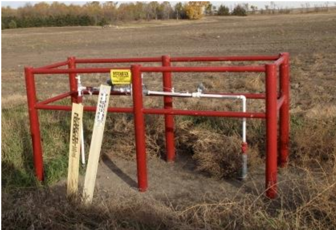
23.) Newest farm tap on system located near Roscoe.
