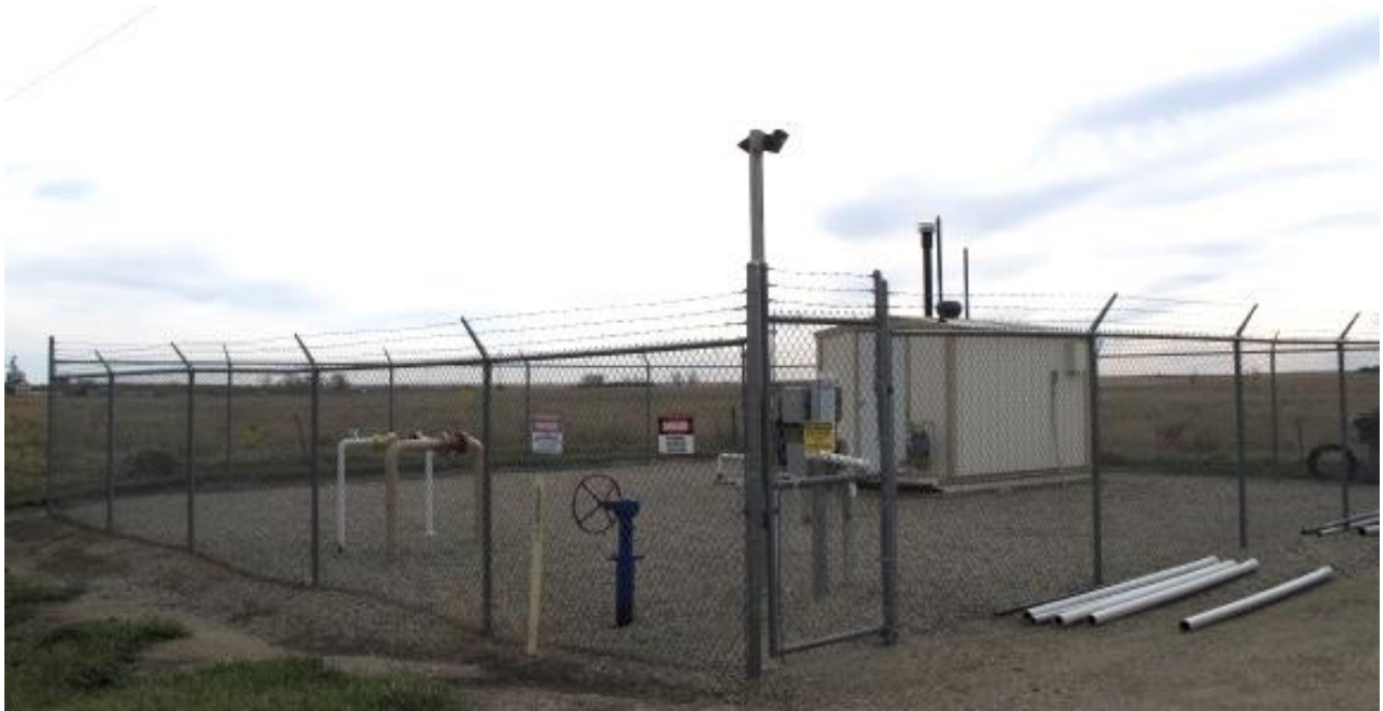
41.) Incoming 3" supplies gas to City of Selby at this tap located near 133 rd Street and 306 th Avenue.
