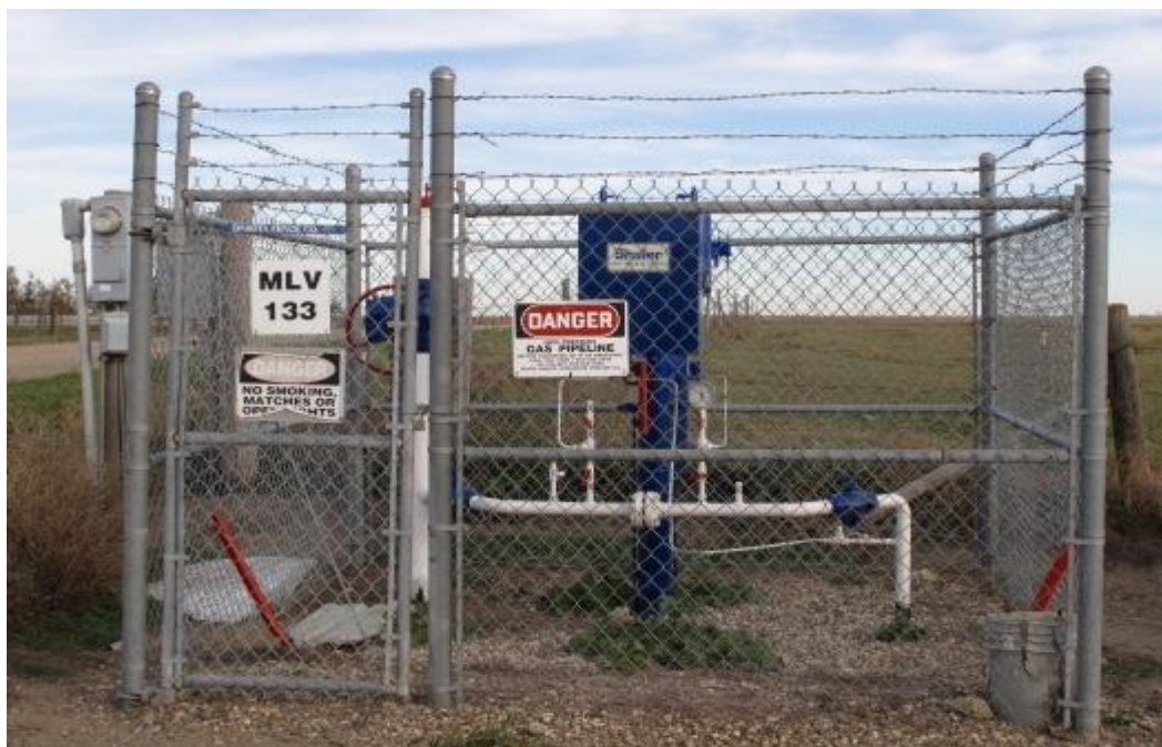
20.) Main line valve and rectifier station at 133 rd Street and 355 th Avenue.
