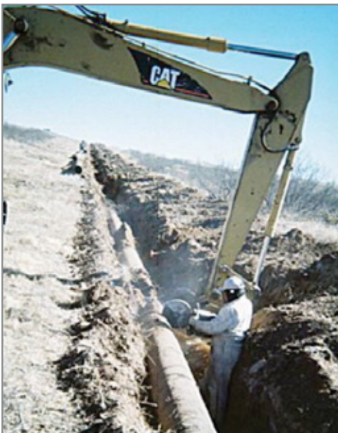
Track hoe lifts pipe to be saw cut. Saws are used instead of torches due to dry grasses in area (fire hazard).
