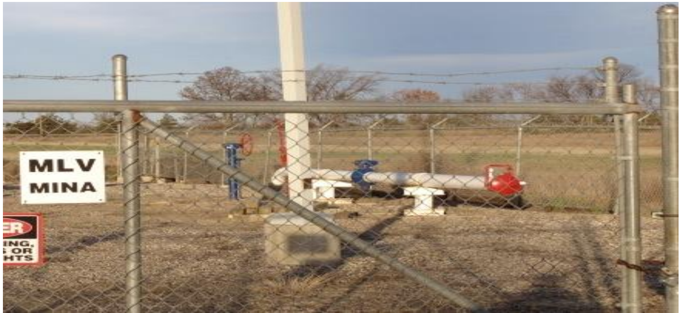
6.) The 8" pig launcher at the kick off MINA Station. There is a 4" intake from Northern Border and the outgoing line is 8" taking the gas to the various points in South Dakota Intrastate Pipeline system.
