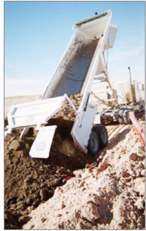
Surface soil from right of way disposed of at landfill.
