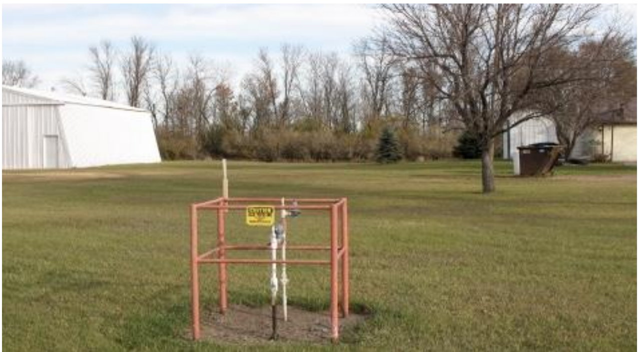
19.) Farm tap on 133 rd Street as Right of Way turns west.
