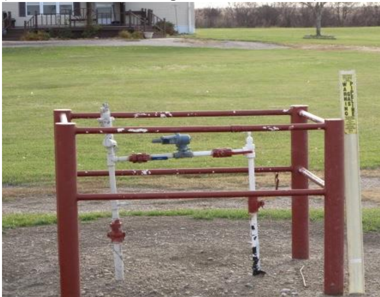
15.) Farm tap serving Montana Dakota Utilities customer at 358 th Avenue near 130 th Street.
