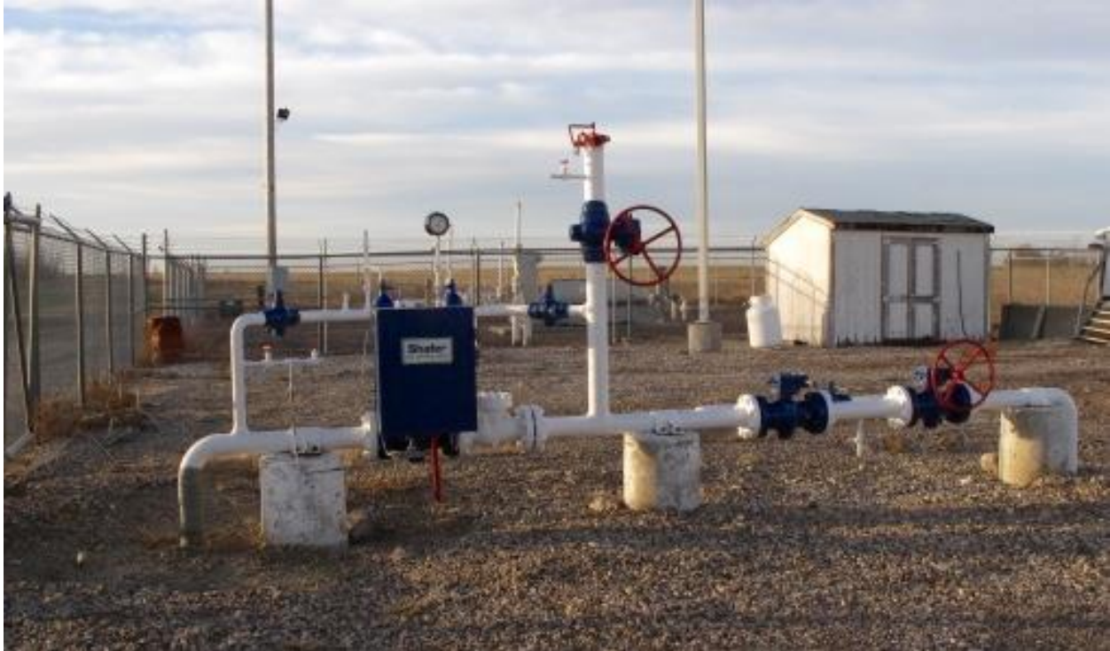
3.) Metering station for MINA. Four Inch line coming into the South Dakota Intrastate MINA station to measure gas coming from the Northern Border Compressor Station a few hundred yards away.
