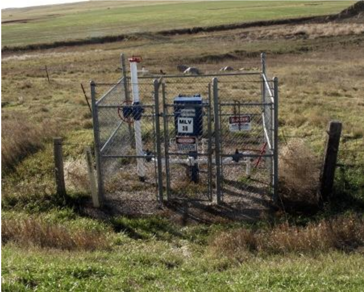
64.) Main Line Valve Station # 36 (for 6" line) on 305 th Avenue.
