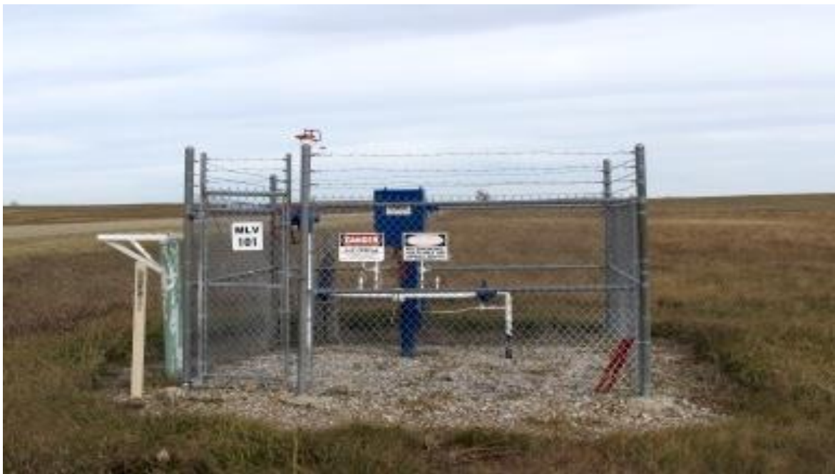
37.) Main line valve station (MLV101) at end of east/west 6". At this point the 6" heads south while the three inch lateral continues west.
