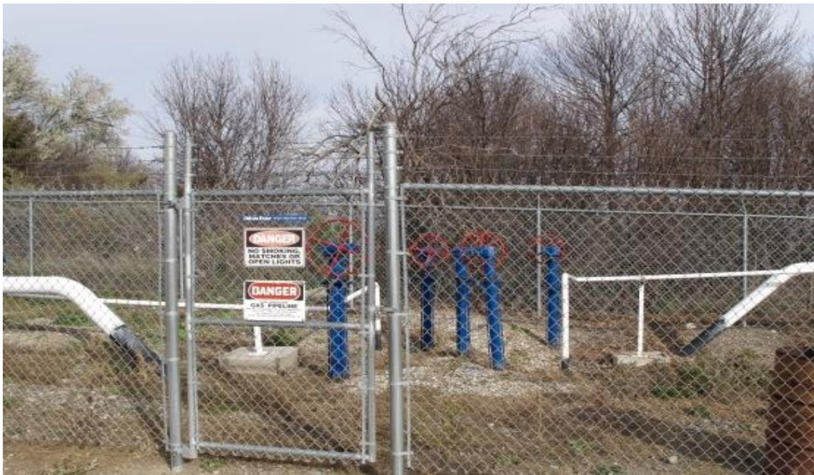
31.) Middle blue valves are crossovers from 8" to 6" with the aforementioned 6" pig launcher on the right and the 8" pig receiver on the left.
