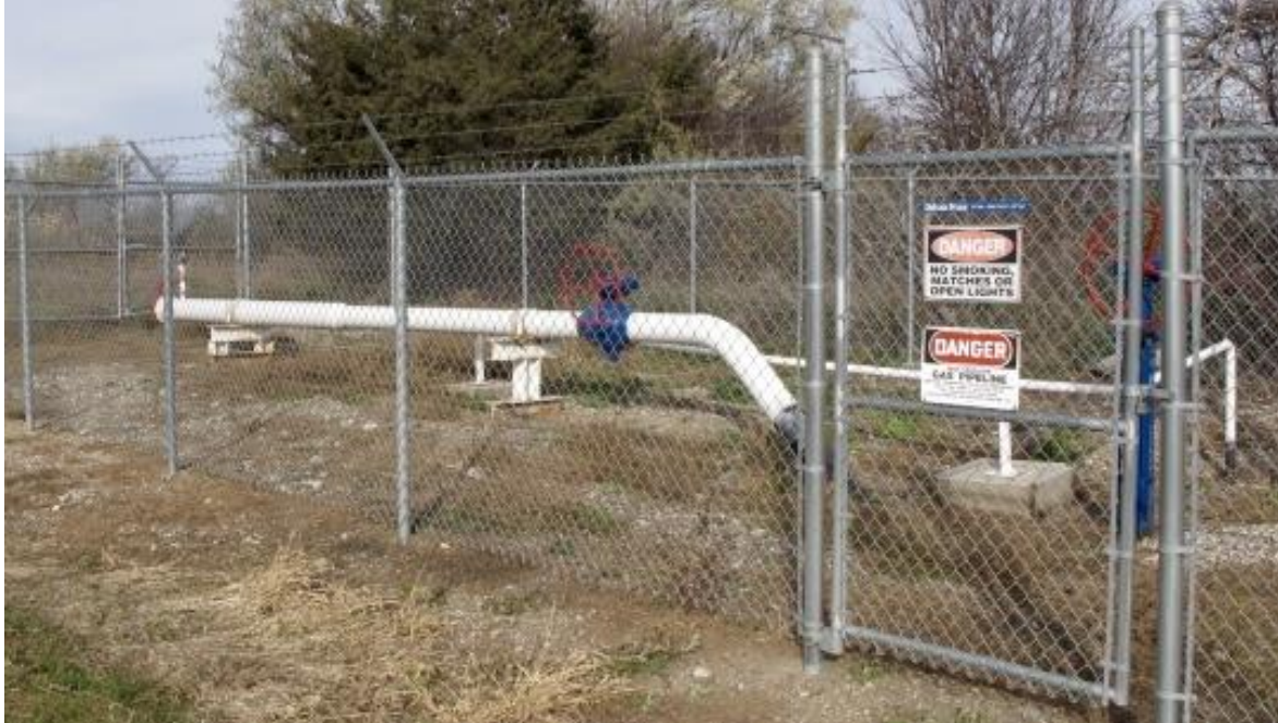
30.) 8" pig receiver at same location coming from kick off of system at Northern Border Compressor station.
