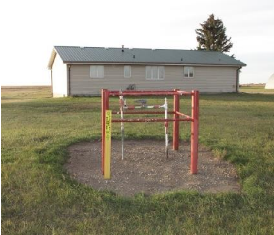
8.) First Farm tap for Montana Dakota Utilities customer approximately five miles from starting point at Mina Station and Northern Border Compressor Station.
