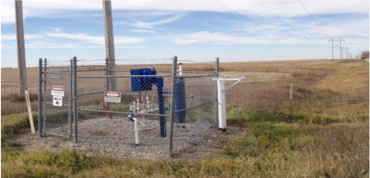
38.) Main Line Valve for 3" lateral heading west. At this point the 6" line from the east turns south toward Pierre.
