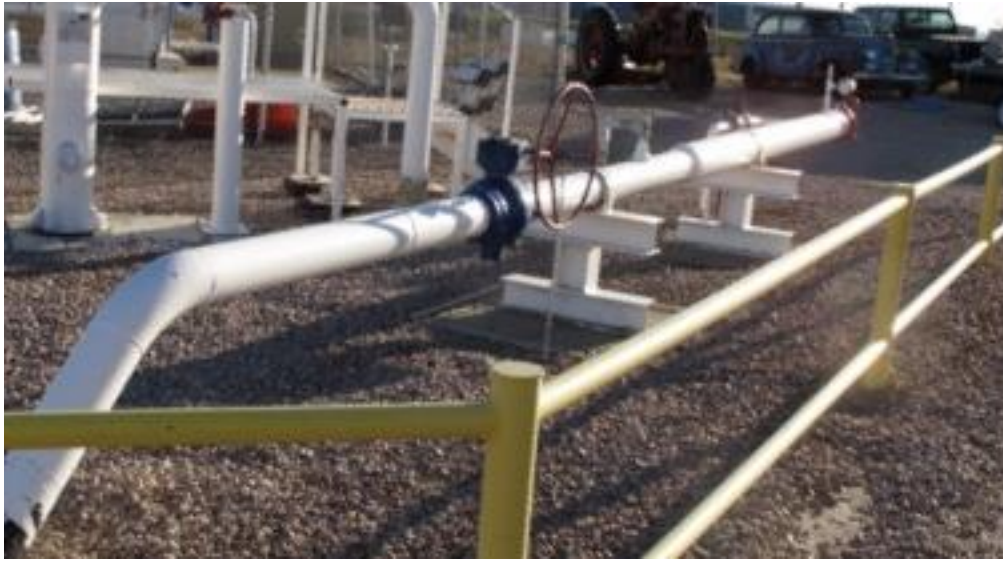
75.) Pig receiver at terminal for 6" line at Pierre.
