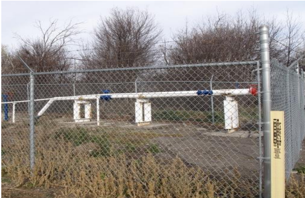
29.) Beginning of 6" line with this 6" pig launcher.
