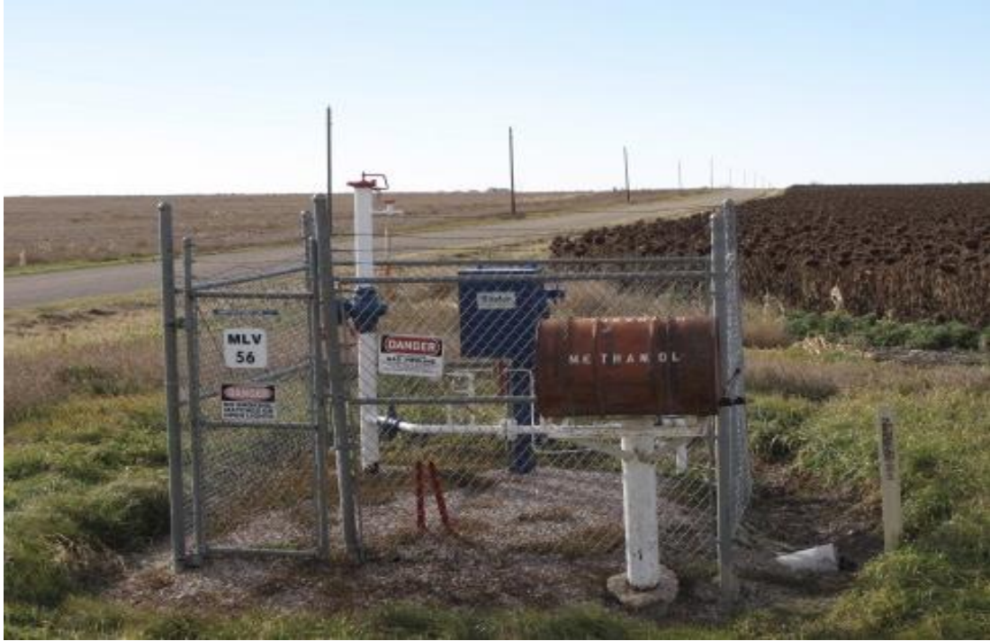
59.) Main Line Valve Station (6") @ 311 th Avenue near 165 th Street.
