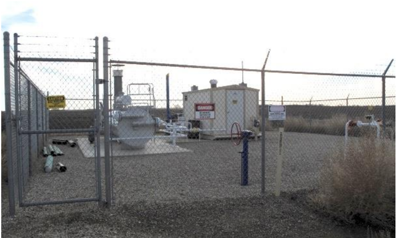
18.) Tap or meter station for City of Ipswich. One of several cities served Montana Dakota Utilities with gas transported by South Dakota Intrastate Pipeline.
