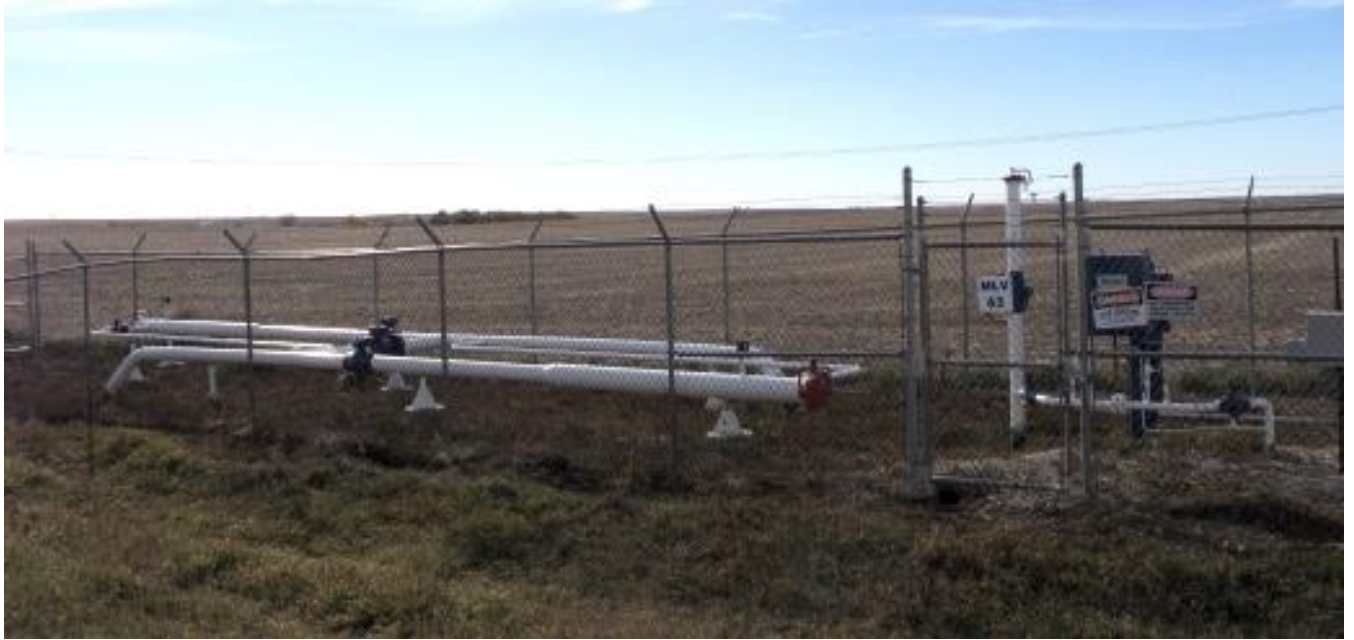
55.) 6" Pigging station with launcher and receiver alongside Main Line Valve Station Number 63. Located on 311 th Avenue.
