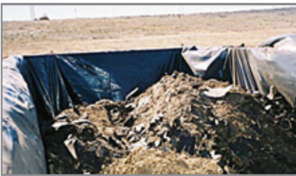
Coating and dirt loaded in lined container for landfill.
