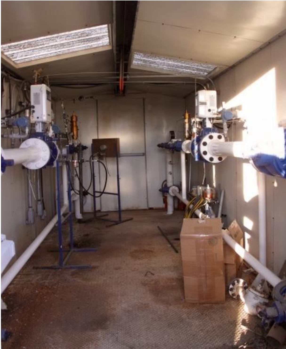
5.) Interior of skid mounted outgoing metering /instrument station at South Dakota Intrastate Pipeline's MINA Station. These meters are mounted inside the skid mounted structure for additional protections from weather or other interference.
