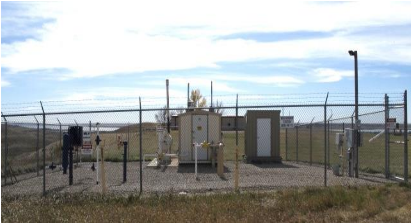
49.) Terminal of Eastbound 3" lateral at City of Mobridge. This is also a tap for City of Mobridge where MDU supplies gas through South Dakota Intrastate Pipeline.
