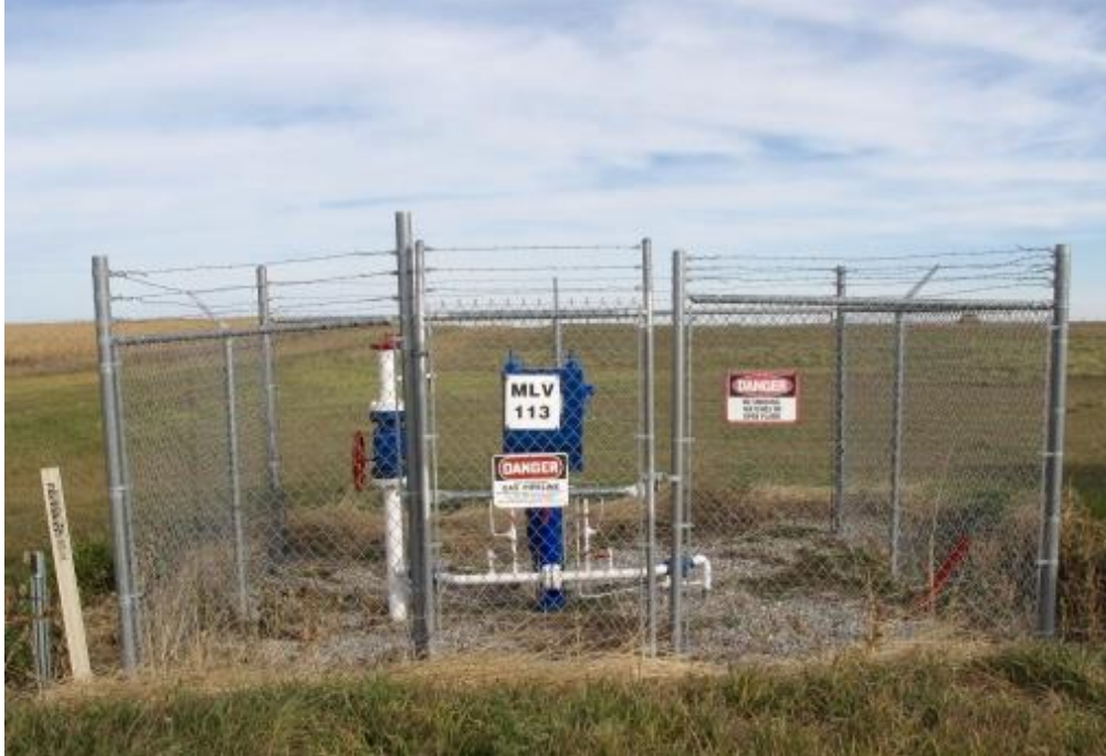
26.) Main Line Valve Station (8") at 334 th Avenue. Pipeline marker on the left appears at one-half mile intervals along the route.
