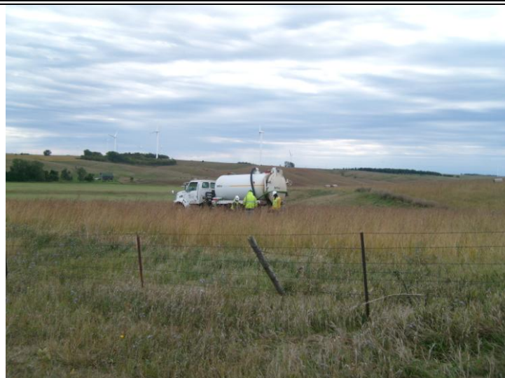
Clean up of the frac-out in the vicinity of Station 558+50.
