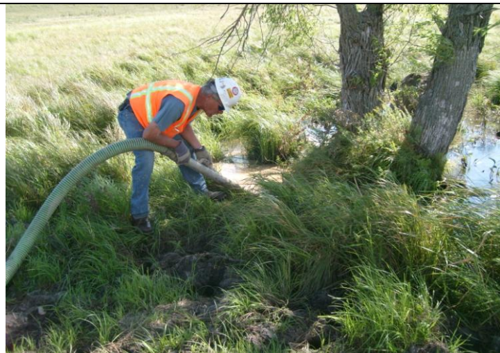
Frac-out in the vicinity of Station 322+20 (east side of ROW).
