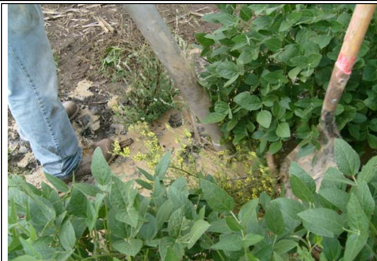
Clean up of frac-out at Station 193+28.
