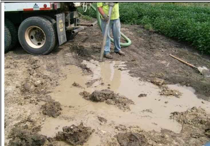
Clean up of frac-out at Station 193+60.
