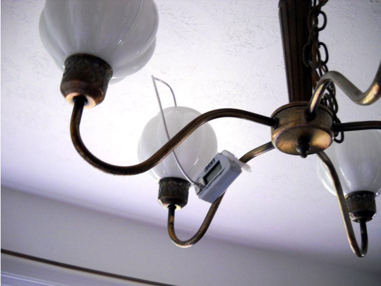
Figure 237: CFL Metering Installation #2
