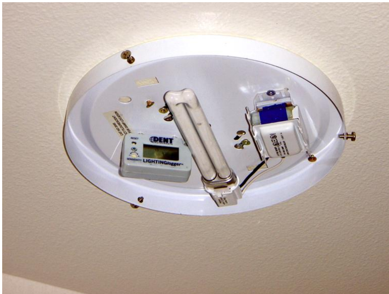
Figure 236: CFL Metering Installation #1
