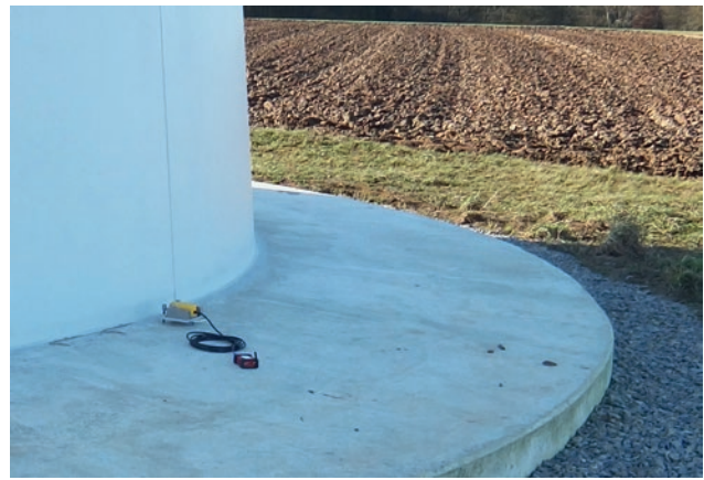
Figure 4.8-1: Vibration measurement point MP A at the tower foundation of WT 5. Photo: Wölfel company
