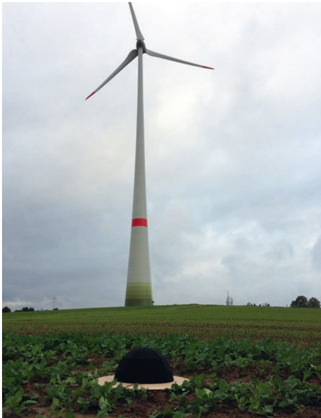
Figure 4.4-1: Wind turbine WT 3 in surroundings used for agricultural purposes. The measurement point with reverberant plate and dual wind screen can be seen in the foreground. Photo: Wölfel company
