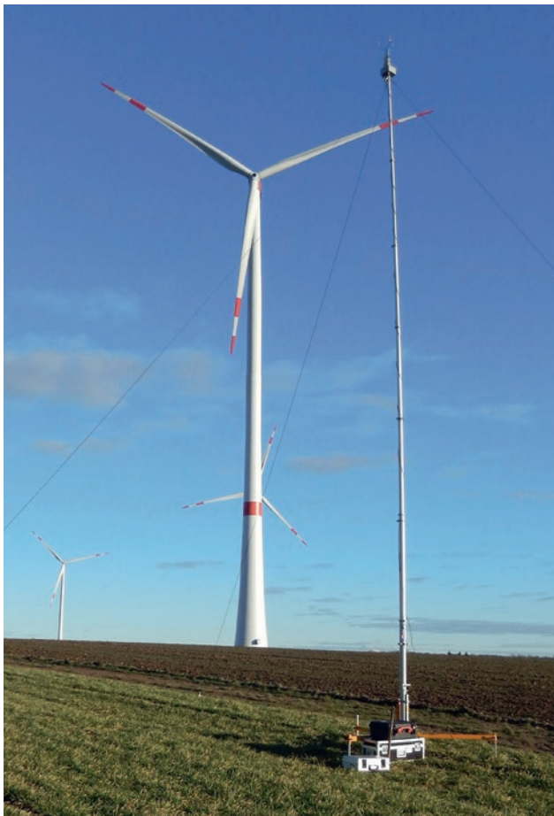
Figure 4.6-1: Wind turbine WT 5 in surroundings used for agricultural purposes. In the foreground you can see the 10 m high wind measurement mast. Photo: Wölfel company
