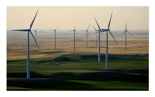
The General Electric 2.82-127 turbine is the primary turbine being considered for the Project.
