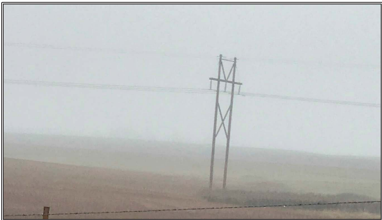
VIEW OF A TYPICAL EXISTING TRANSMISSION LINE
