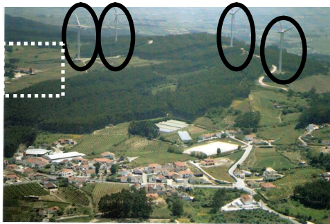
Figure 1. Aerial view of the WT home of Family R., isolated on upper left (dashed square) with the four wind turbines nearby (ovals).
