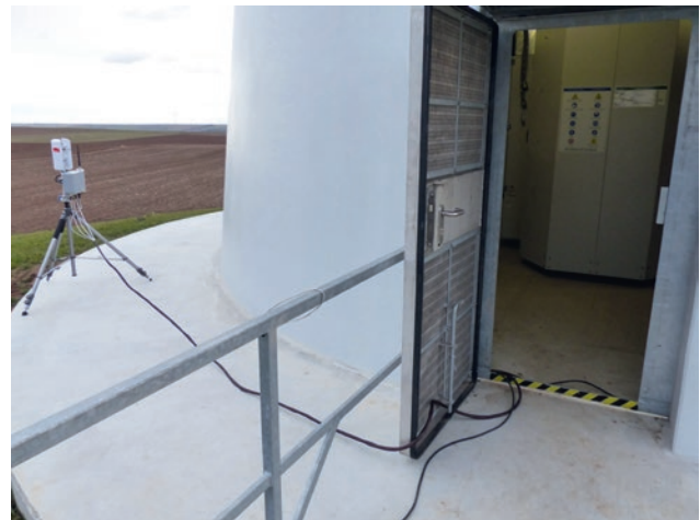
Figure 4.5-5: Data is constantly collected inside the system during the measurement and transmitted by radio (left). Photo: LUBW
