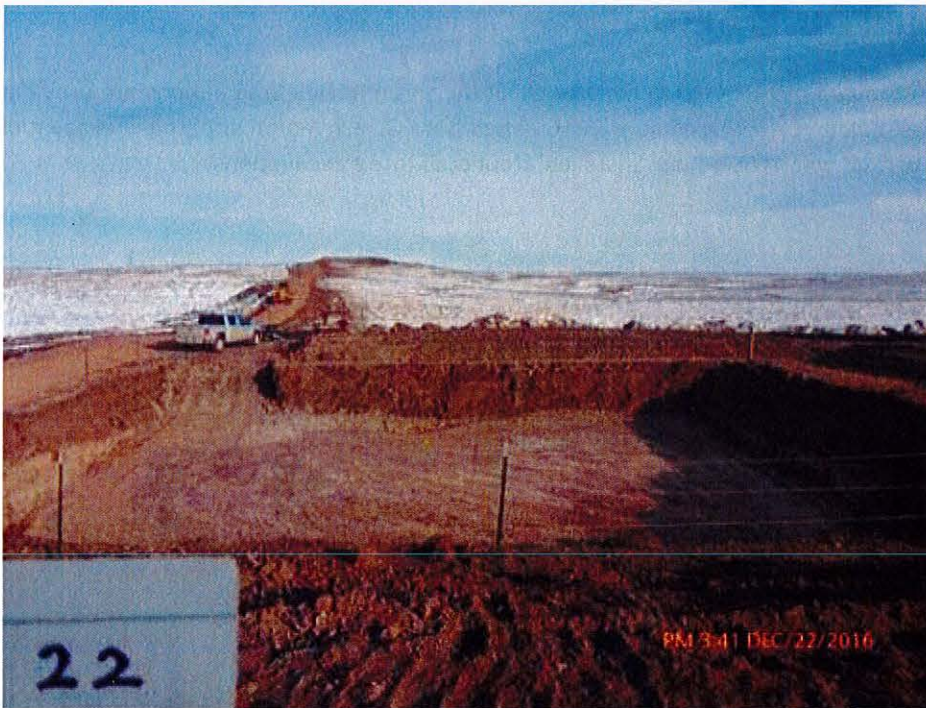
Figure 6 Excavation at turbine T22
