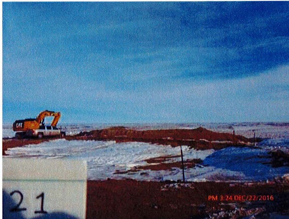
Figure 1 Excavator near T21
