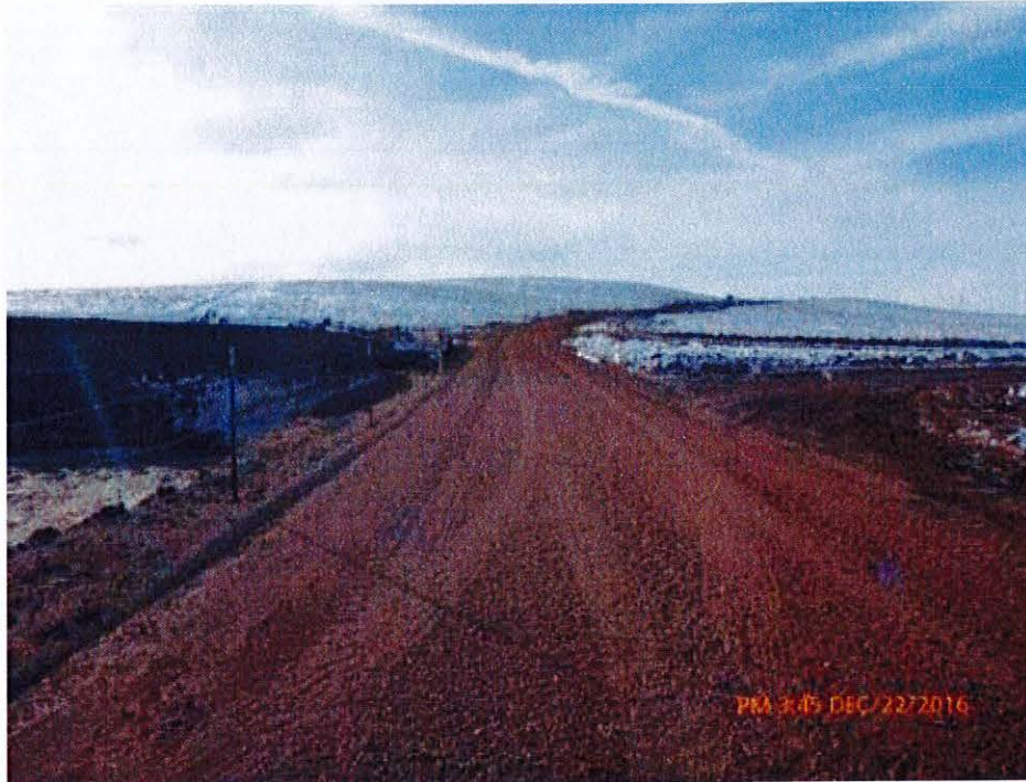
Figure 4 Turbine access road near T23
