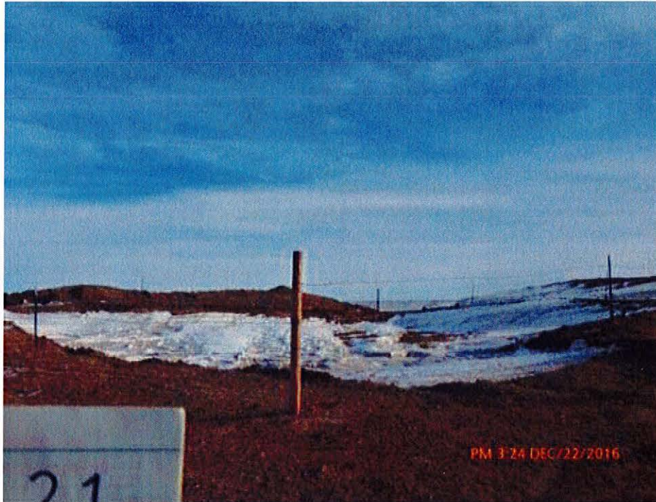
Figure 5 Excavation at turbine T21
