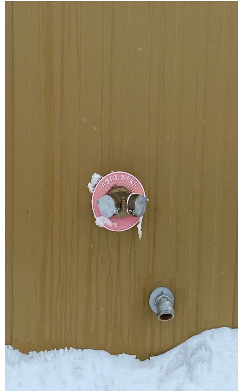
Southeast corner of Maintenance Building
