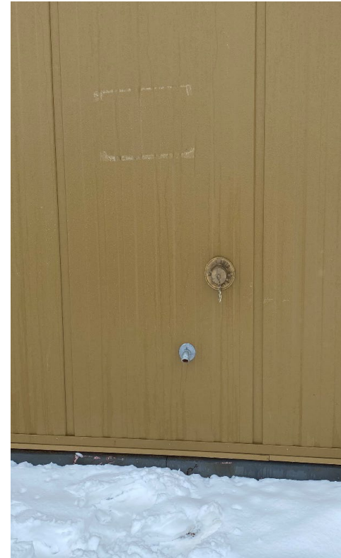
North side of Admin Building
