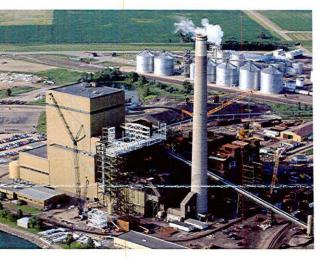
Construction of the new air-quality control system (AQCS) at Big Stone Plant is more than 50 percent complete. When finished, the AQCS will reduce the plant's nitrogen oxide, sulfur dioxide, particulate matter, and mercury emissions by 80 to 90 percent. These environmental upgrades will help Big Stone Plant meet federal regulations, including new mercury standards and regulations to reduce haze.
