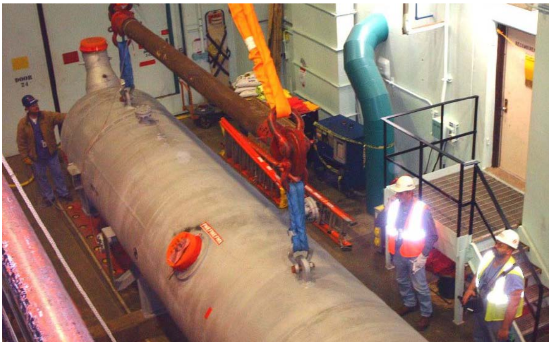
Feedwater Heater 15A on Turbine Deck
