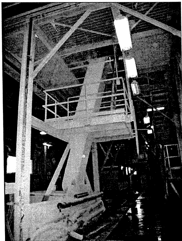
Figure 6 - SDA Hopper Ash Chute.
