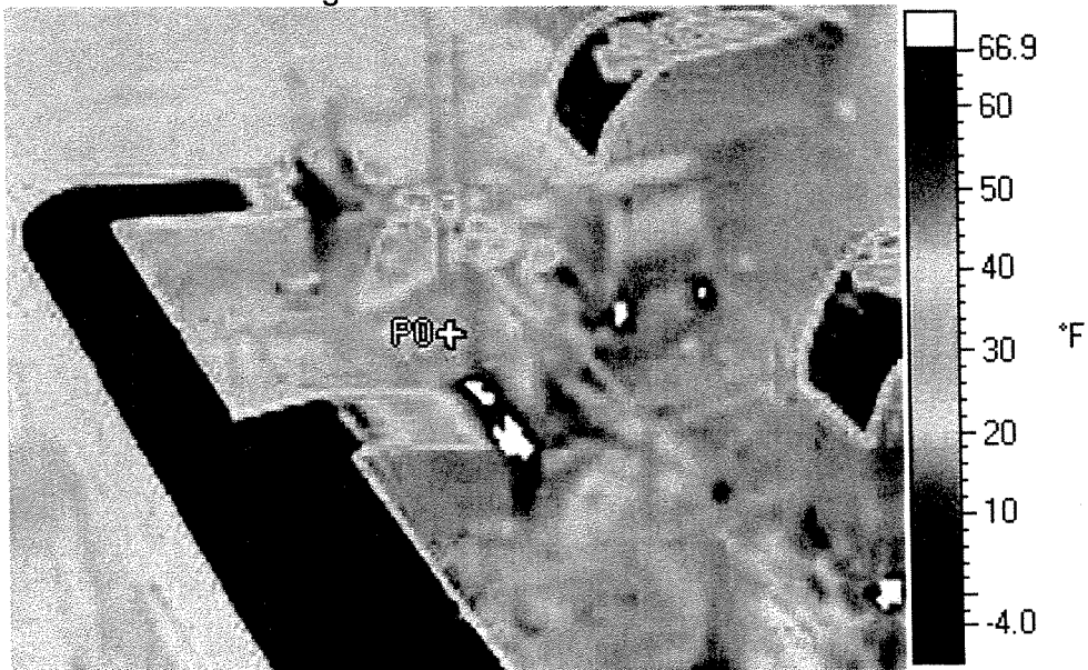
Figure 8 – SDA Outlet IR View.
