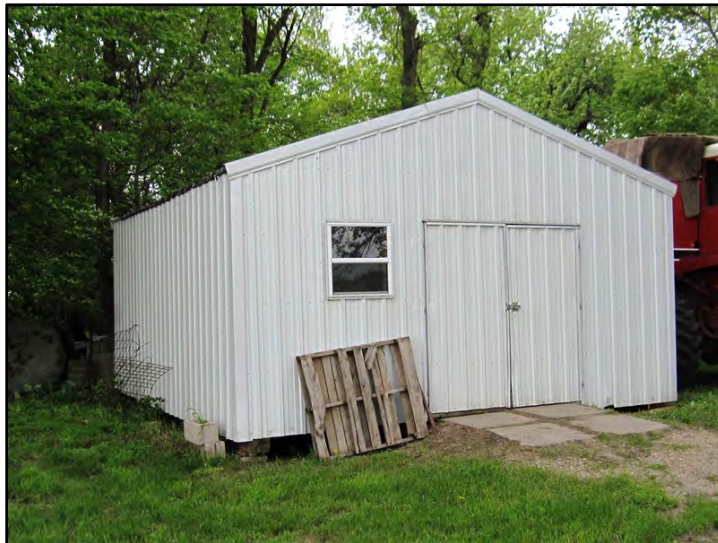
Figure 3–39. View to northwest of Building 6 east primary façade and south elevation.
