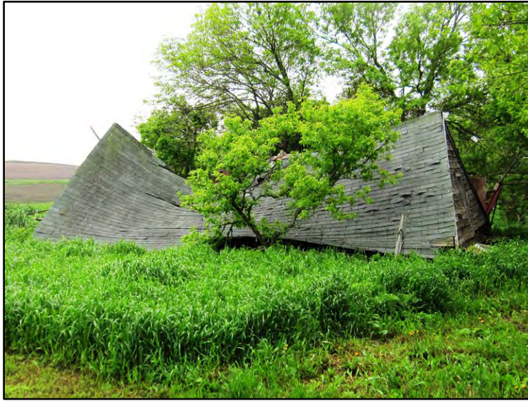
Figure 3–96. View to east of collapsed barn Building 3.
