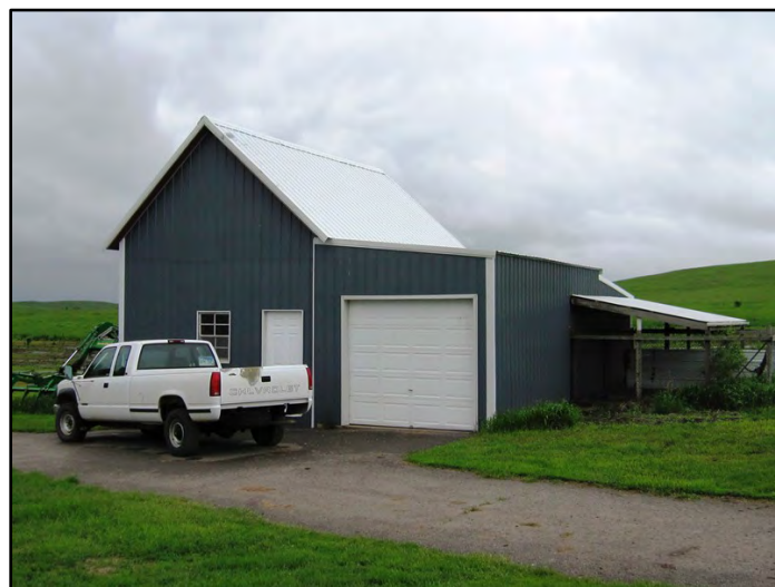
Figure 3–7. View to southwest of Building 4 garage east primary façade and north elevation.
