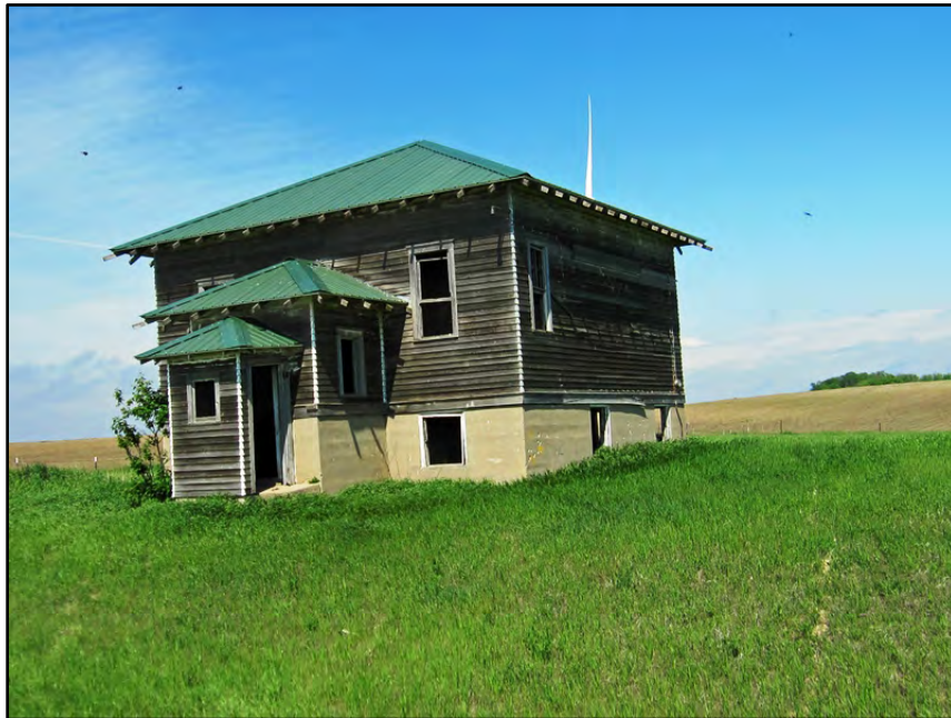
Figure 3–3. View to northeast of schoolhouse/meeting hall Building 1 west primary façade and south elevation.
