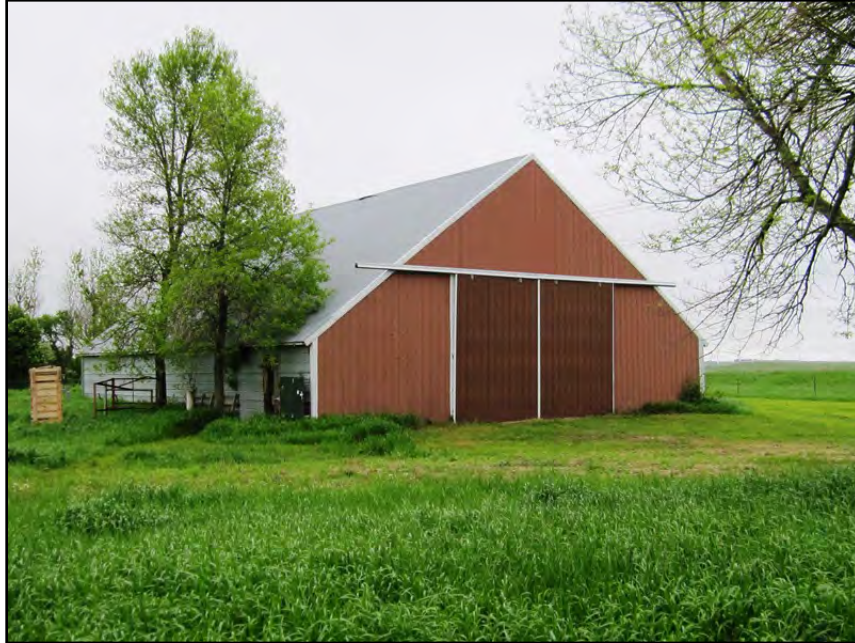
Figure 4–2. view to north of historic age machine shed.
