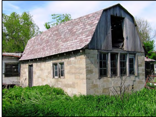
Figure 3–78. View to northeast of dairy barn Building 6 west primary façade and south elevation.
