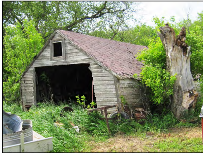
Figure 3–85. View to northwest of Building 2 south primary façade and east elevation.
