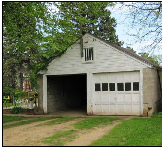
Figure 3–48. View to northeast of garage Building 2 west primary façade and south elevation.
