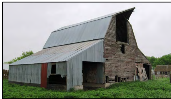
Figure 3–116. View to northwest of Building 6 east primary façade and south elevation.
