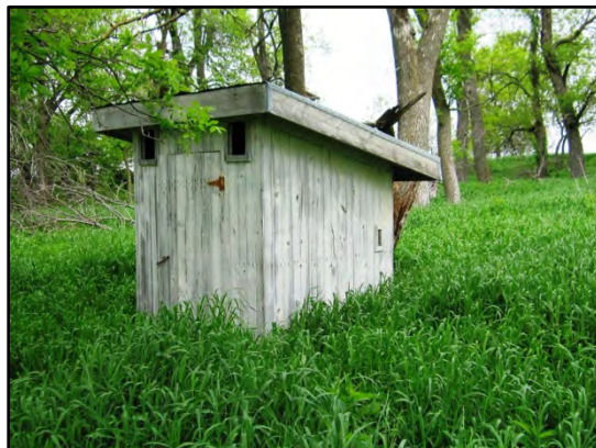
Figure 3–120. View to northeast of pump house Building 5 west primary façade and south elevation.
