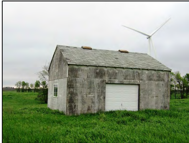
Figure 3-109. View to northeast of Building 11 south primary façade and west elevation.
