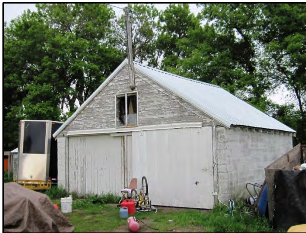
Figure 3–100. View to southwest of storage Building 2 east primary façade and north elevation.
