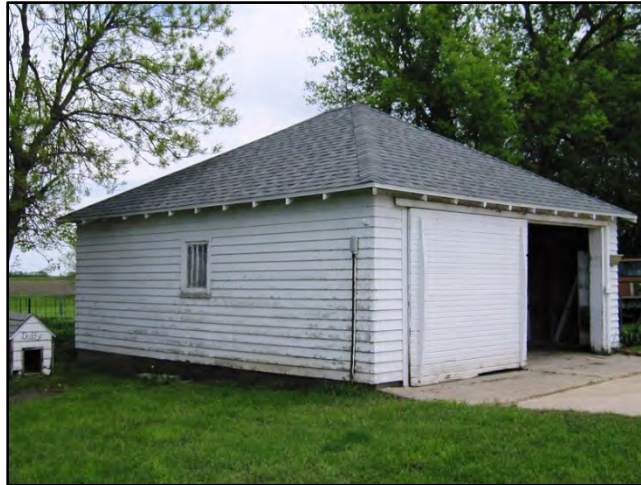
Figure 3–64. View to southeast of garage Building 3 west primary façade and north elevation.
