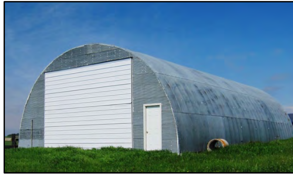
Figure 3–1. View to northeast of Building 1 Quonset hut west primary façade and south elevation.
