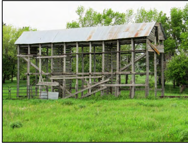
Figure 3-108. View to northwest of Building 10 south and east elevations.
