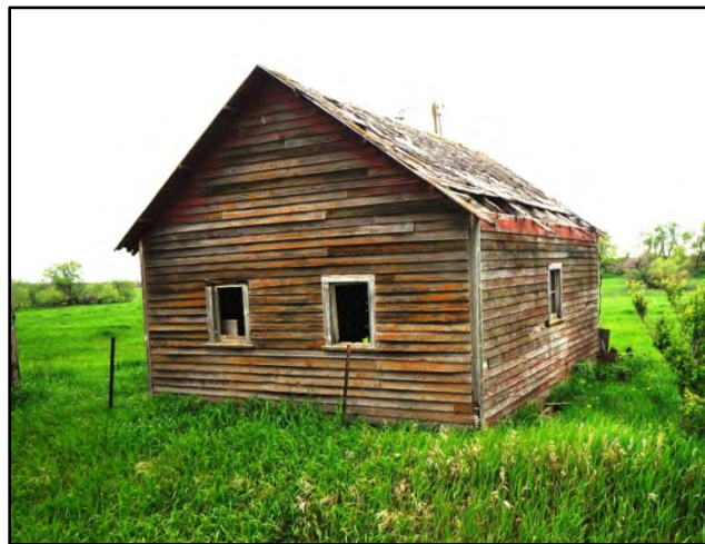
Figure 3–31. View to southeast of historic age residence north and east elevations.
