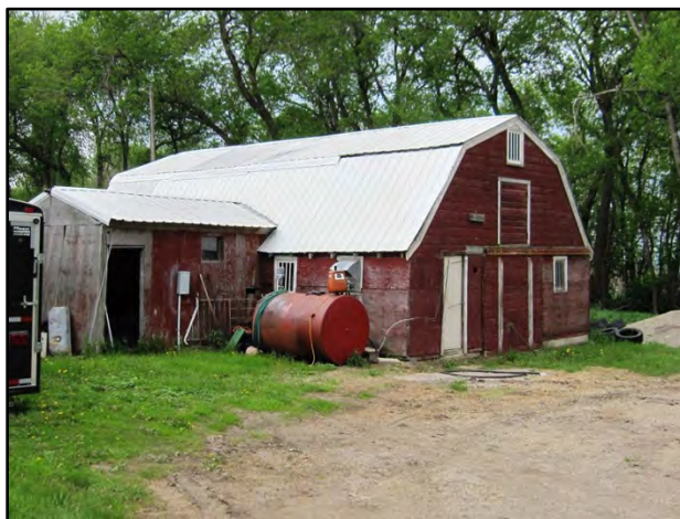
Figure 3–125. View to northwest of Building 7 east primary façade and south elevation.
