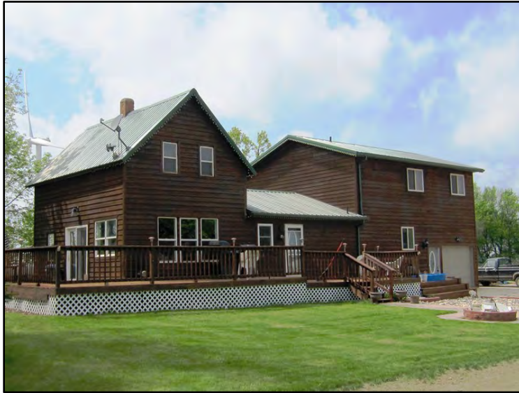
Figure 3–15. View to northwest of Building 1 residence east and south elevations. The portion on the left is the original farmhouse, and the two segments to the right are modern additions.
