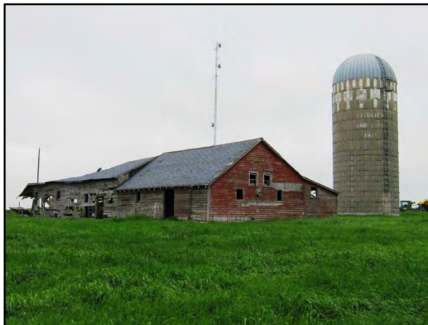
Figure 3–30. View to southwest of barn (Building 1) north primary façade and east elevation, and concrete stave silo constructed in 1965 by Diedrich and Sons.
