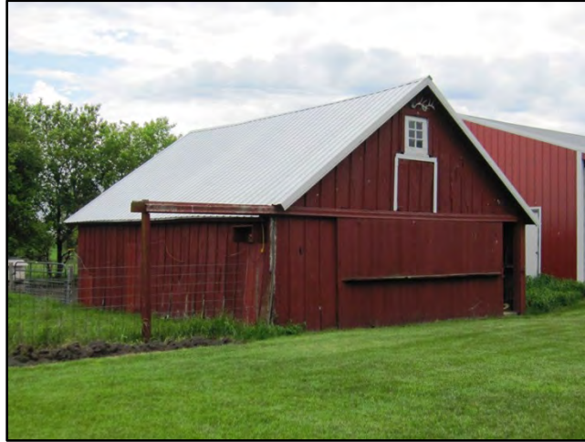
Figure 3–52. View to southwest of machine shed Building 7 north primary façade and east elevation.
