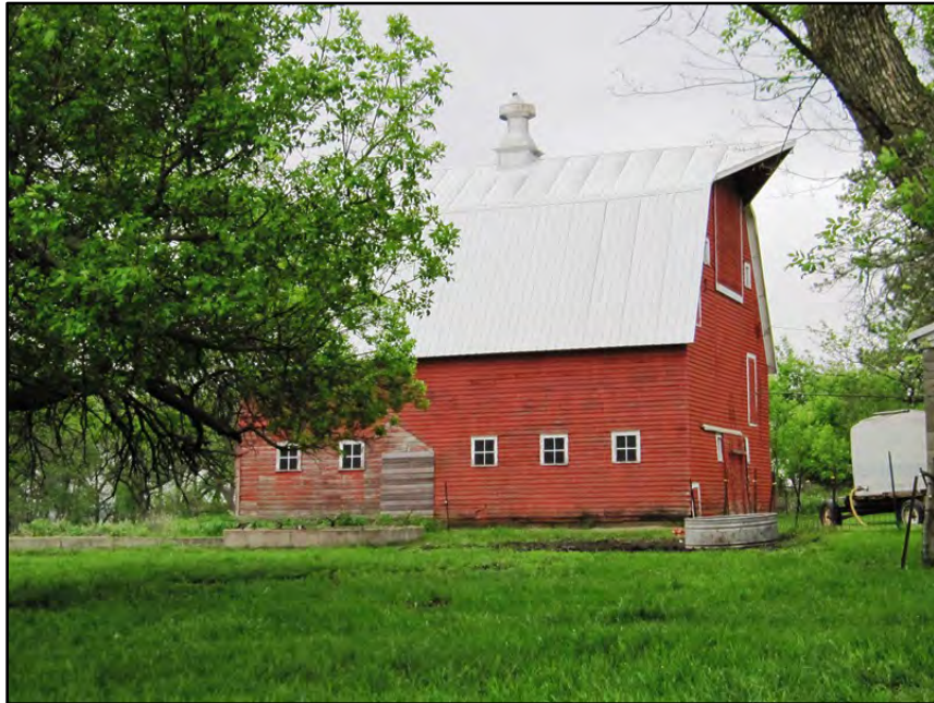
Figure 3–55. View to east of Hexem Barn south primary façade and west elevation. The circular outline in the foreground on the left from a demolished silo. Note the outline on the barn wall of the silage chopper house that is no longer extant.
