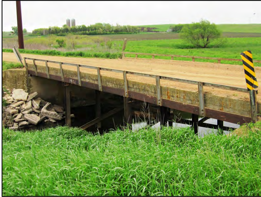
Figure 4-5. view to southeast of 207 th Street Bridge.
