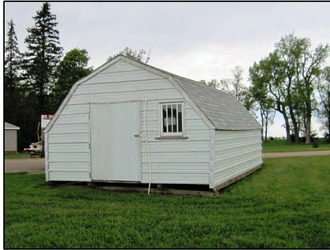
Figure 3–36. View to northwest of Building 3 south primary façade and east elevation.
