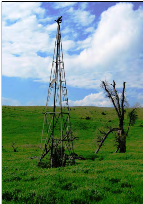
Figure 3–23. View to north of windmill with missing vane.
