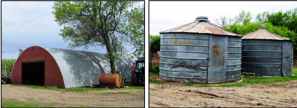
Figure 2–16. Site BK00001244 has example of twentieth century prefabricated buildings and structures. The Quonset hut on the left is a Post-World War II building form. The grain bins on the right are older than most in the study area, based on the material and fabrication techniques.
