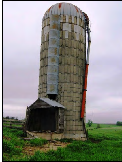
Figure 3–106. View to north of Building 8 silo and silage chopper house, with silage blower tube on left.
