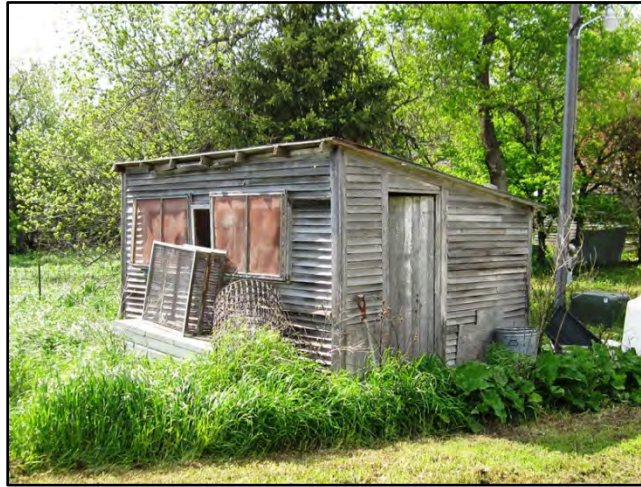
Figure 3–76. View to southwest of chicken coop Building 3 east primary façade and north elevation.
