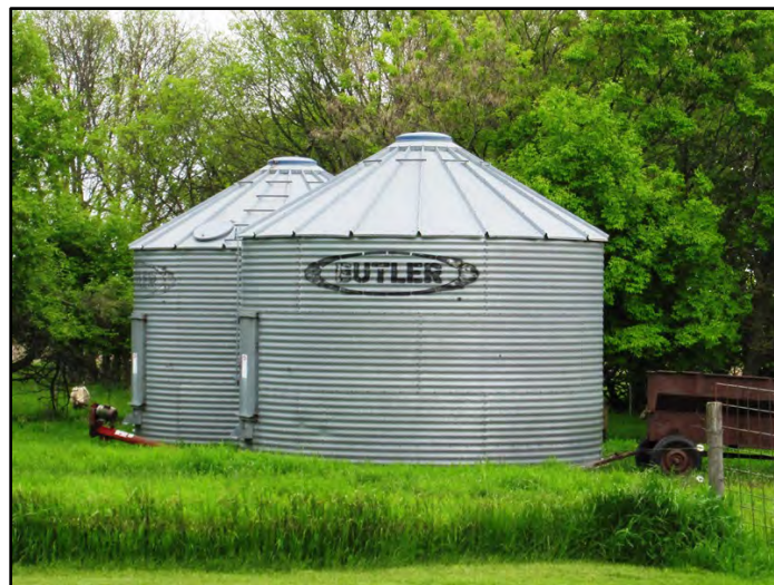
Figure 3–51. View to east of Building 6, two modern age Butler grain bins.
