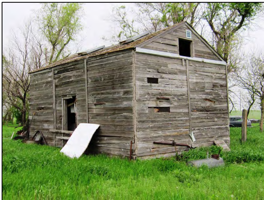
Figure 3–21. View to northwest of Stansky farm granary south primary façade and east elevation.
