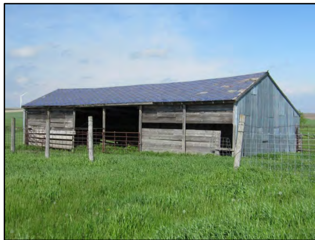
Figure 3–2. View to northeast of feed shed Building 2 west primary façade and south elevation.
