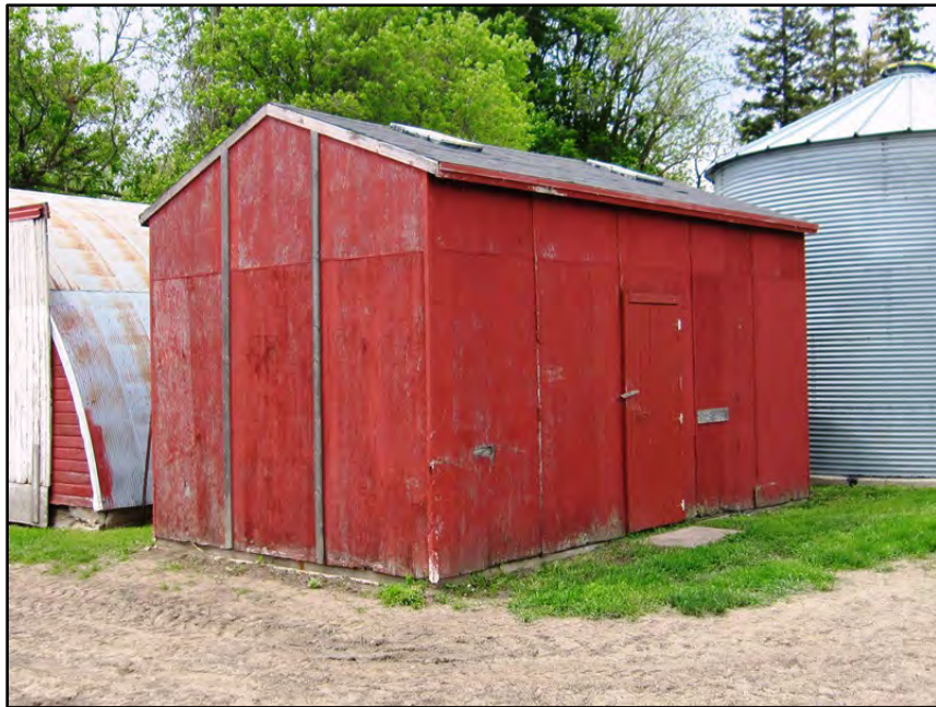
Figure 3–41. View to northwest of Building 8 east façade and south elevation.
