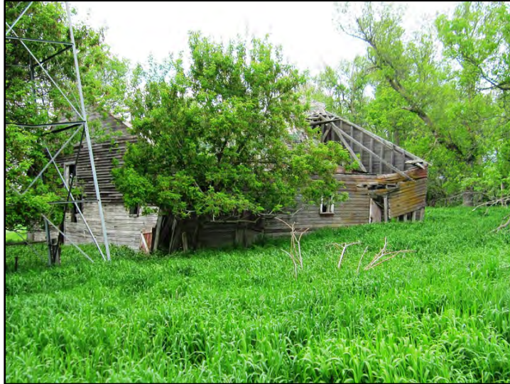
Figure 3–121. View to northwest of Building 6.
