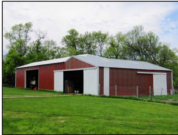
Figure 3–67. View to northwest of Building 6 machine shed south primary façade and east elevation.
