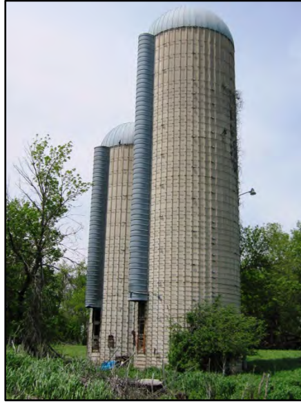
Figure 3–69. View to north of Building 2 Midtounse concrete stave silos south and west elevations.
