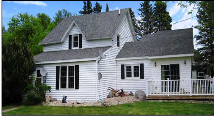
Figure 3–47. View to northeast of residence west primary façade (Building 1). The original building core is located on the left-rear. The shed roof segment on the left foreground and portion to the right are additions.
