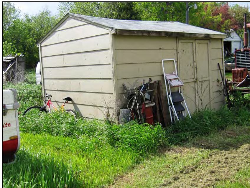
Figure 3–81. View to northwest of Building 10 east primary façade and south elevation.
