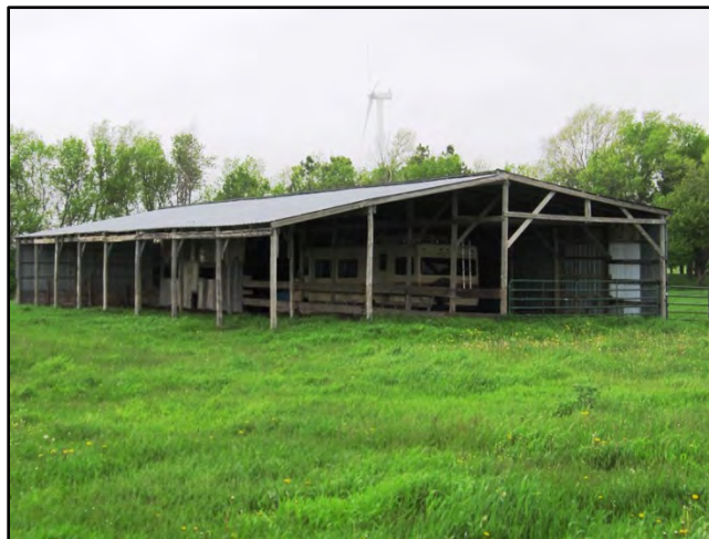
Figure 3–107. View to northwest of pole barn Building 9.
