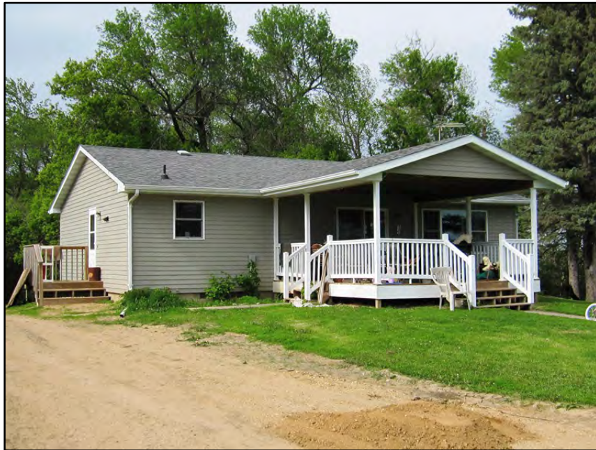
Figure 3–84. View to north of Building 1 modern residence south primary façade and west elevation.
