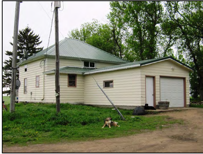
Figure 3–99. View to southeast of residence Building 1 north and west elevations. The original first floor mudroom is located in the corner on the left.
