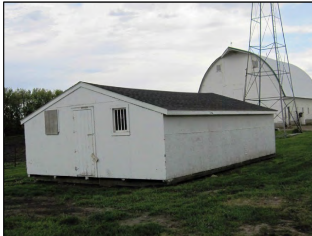
Figure 3–37. View to southeast of Building 4 north primary façade and west elevation.
