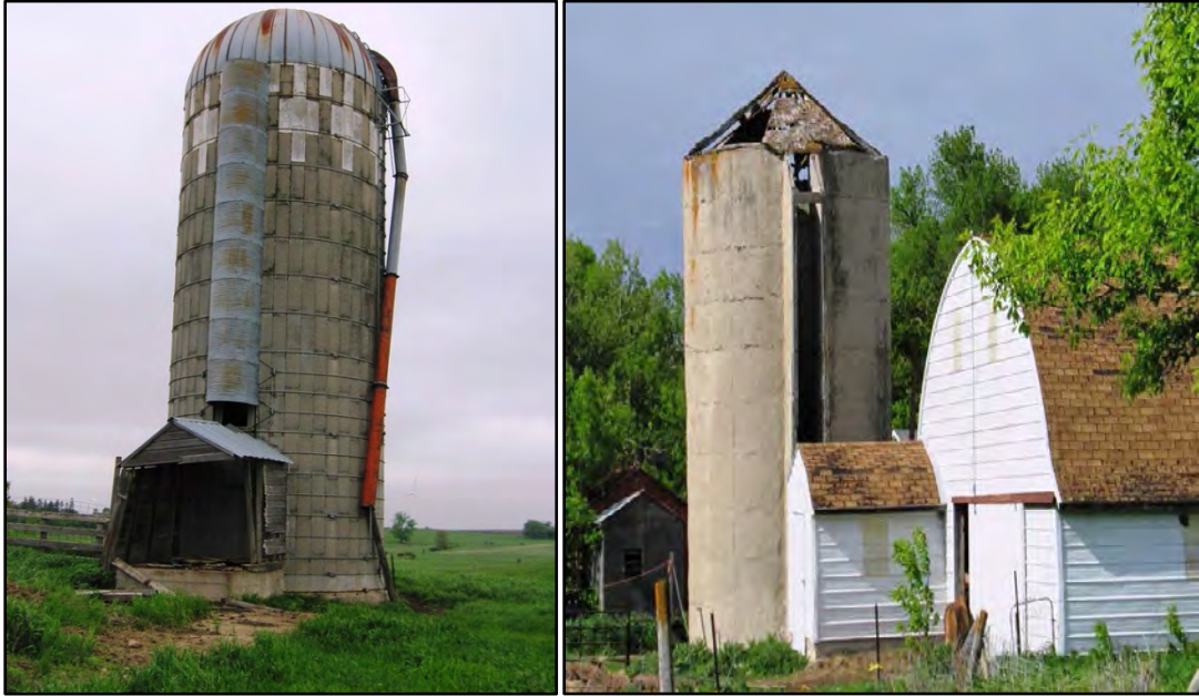
Figure 2–15. The concrete stave silo on the left is located at site BK000001395. It has an intact assemblage of a silage blower (red, on left), silo, silage housing and silage chopper house. Diedrich & Sons constructed many study area concrete stave silos in the mid-1960s. The poured concrete silo on the left is at site BK000001350 and has an unusual vernacular design.
