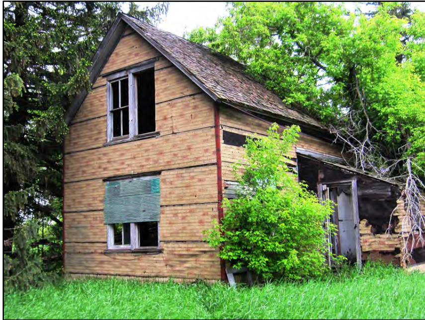
Figure 3–110. View to northwest of Building 1 south and east elevations.
