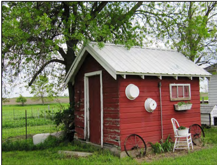
Figure 3–65. View to east of pump house Building 4 north primary façade and west elevation.
