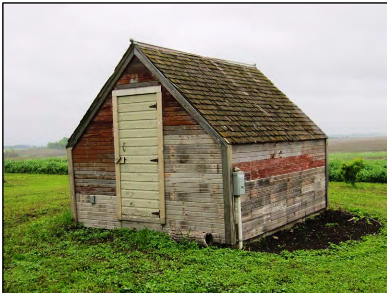
Figure 3–97. View to northeast of outbuilding Building 4 west primary façade and south elevation.
