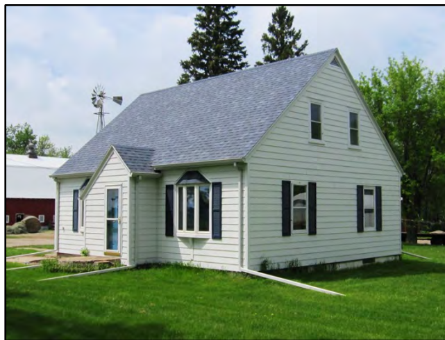
Figure 3–123. View to northwest of Building 1 south primary façade and east elevation.
