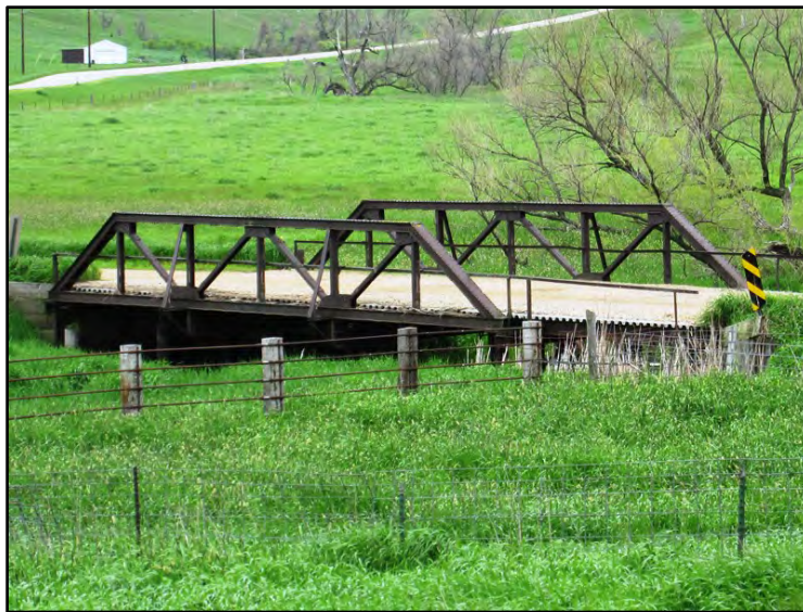
Figure 2–4. Site BK00002198/BK00000185 is a Warren pony truss bridge constructed in 1910 and then later relocated to the Richland Township on 206 th Street for the east branch of the Deer Creek crossing.
