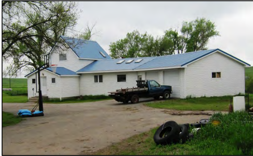
Figure 3–13. View to southwest of historic age residence Building 5 east primary façade and north elevation. The original farmhouse is the two-story segment on the left. The remaining portions are additions.
