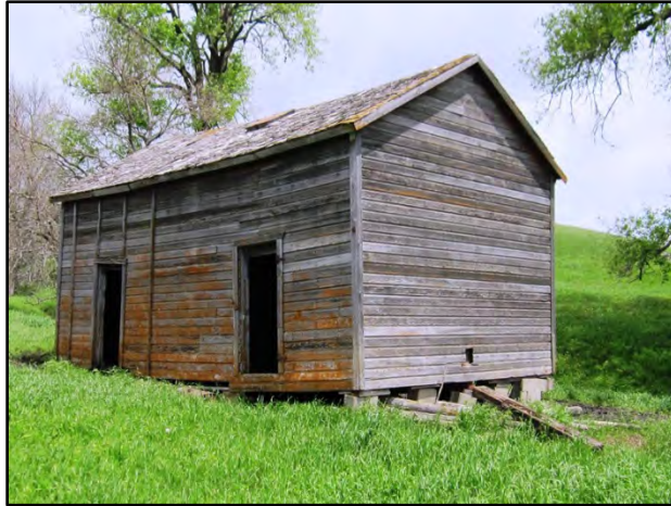
Figure 3–28. View to northeast of granary Building 2 west primary façade and south elevation.
