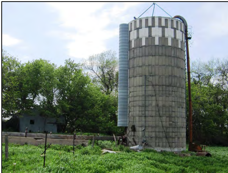
Figure 3–90. View to west of Building 5 concrete stave silo associated with demolished barn (note foundations on left). The red silage blower is located on the right. The collapsing Building 6 is in the left, rear.
