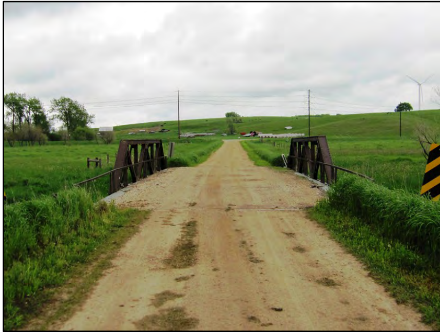
Figure 4–6. View to east of 206 th Street Bridge over east branch of Deer Creek.
