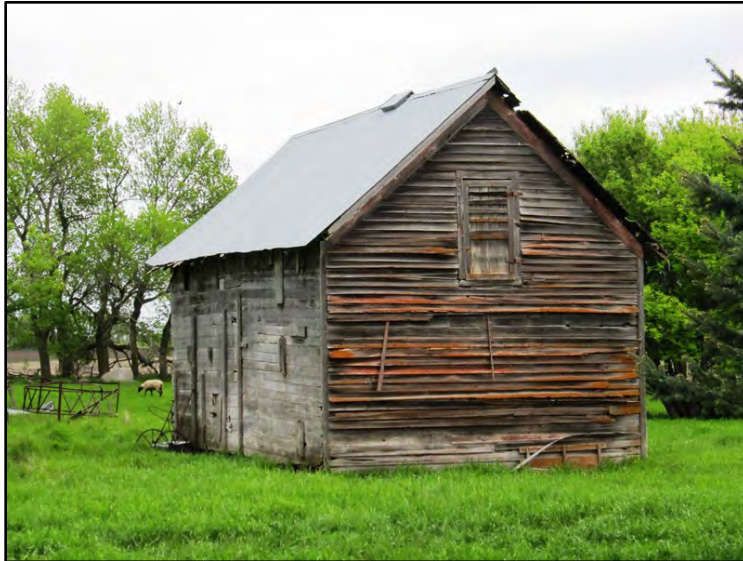
Figure 3–50. View to southeast of granary Building 4 west and north elevations.
