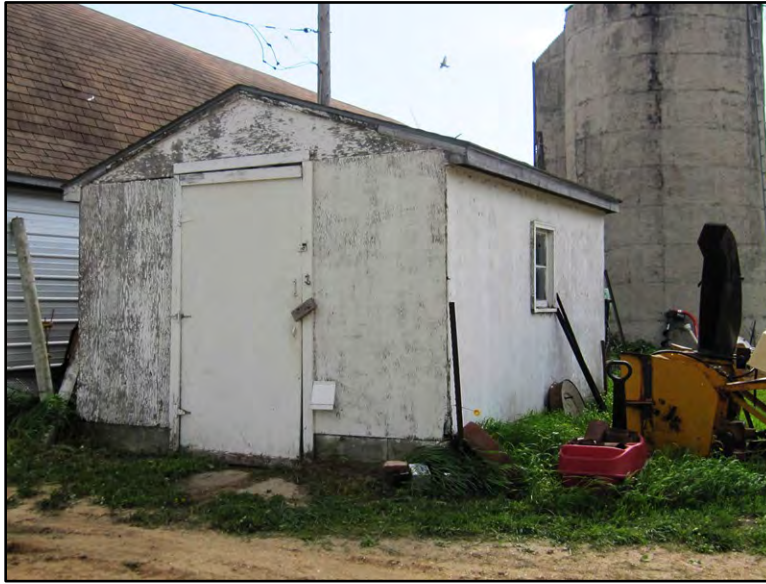
Figure 3–89. View to west of modern storage shed on northeast side of Quonset barn that forms part of the Building 4 complex.
