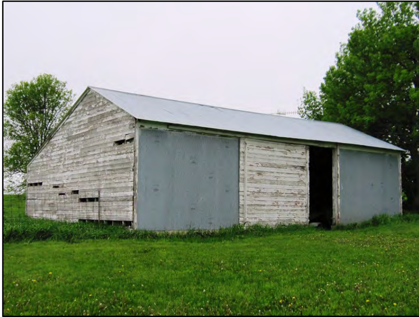
Figure 3-105. View to southwest of Building 7 north primary façade and east elevation.
