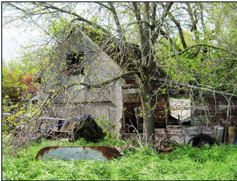
Figure 3–83. View to northwest of granary Building 12 south elevation.
