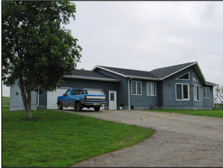
Figure 3–6. View to northeast of Building 3 modern residence south primary façade and west elevation.
