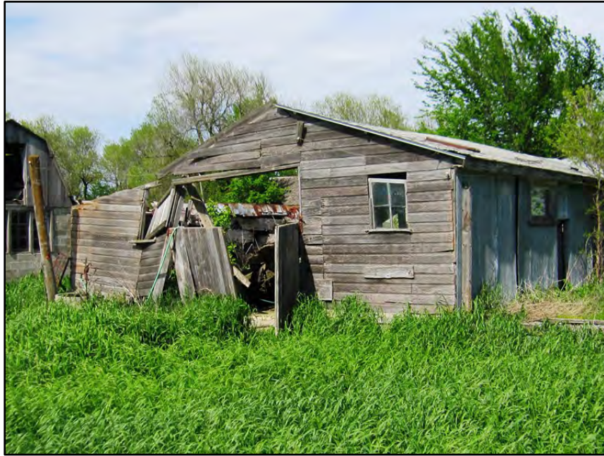
Figure 3–80. View to south of Building 8.
