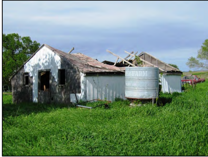
Figure 3–91. View to northeast of Building 7 west façade and south elevation.
