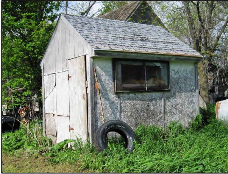
Figure 3–82. View to northeast of storage Building 11 west primary facade and south elevation.
