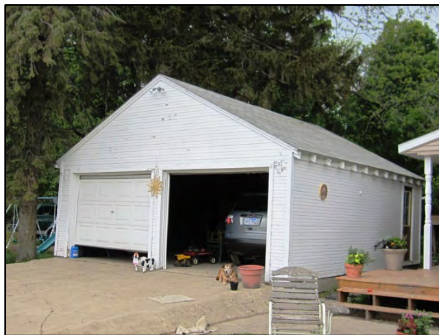
Figure 3–34. View to southwest of garage (Building 1) east primary façade and north elevation.
