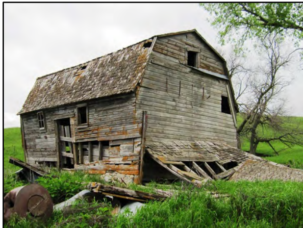
Figure 3–29. Wisconsin style dairy barn south primary façade and east elevation.
