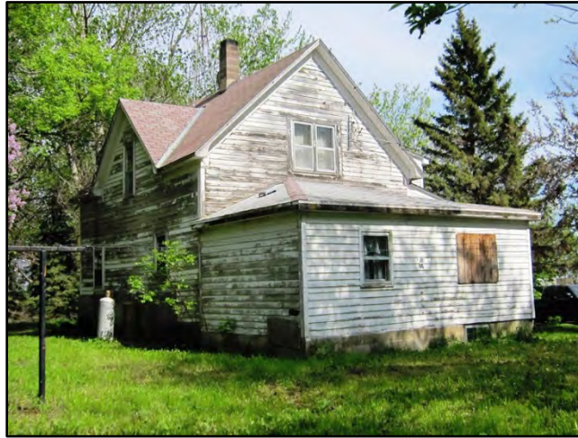
Figure 3–74. View to southeast of residence Building 1 west and north elevations.
