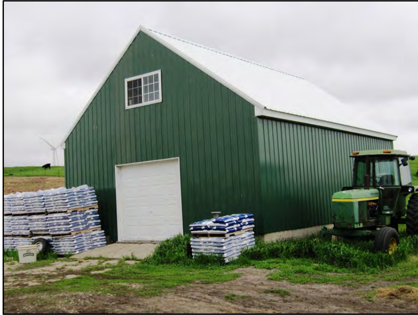
Figure 3–9. View to southeast of historic age machine shed Building 1 north primary façade and west elevation.
