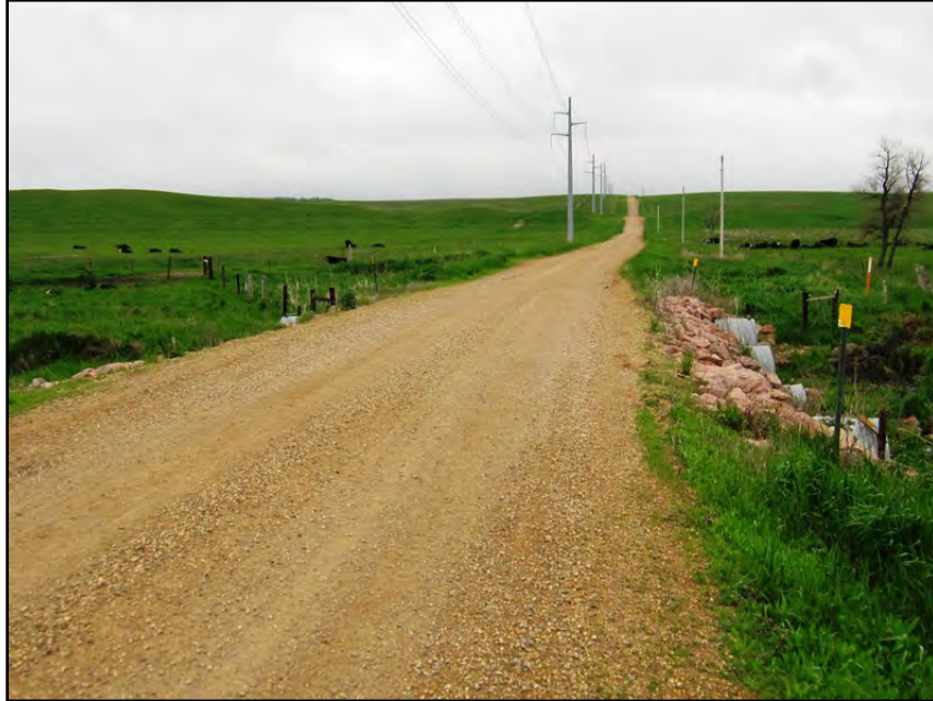
Figure 4–4. View to south of former 484 th Avenue Bridge site.
