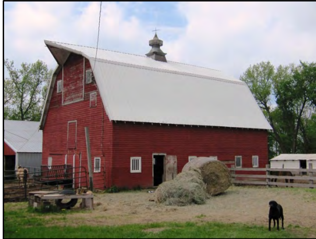
Figure 3–124. View to northwest of Building 3 barn south primary façade and east elevation.
