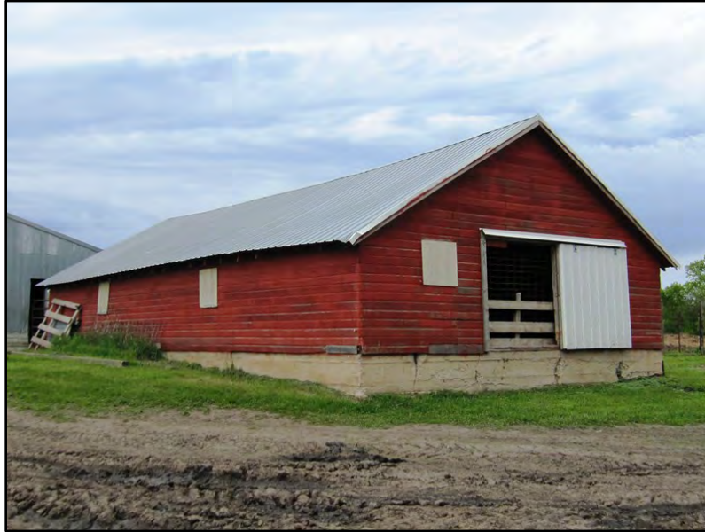
Figure 3–44. View to northeast of feed barn (Building 11) south primary façade and west elevation.
