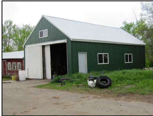
Figure 3–11. View to northwest of modern garage Building 3 south primary façade and east elevation.
