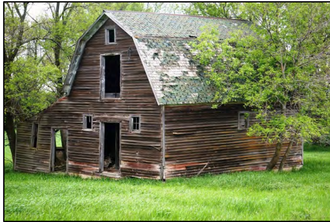
Figure 3–32. View to northwest of historic age barn (east) Building 2 east primary façade and north elevation.
