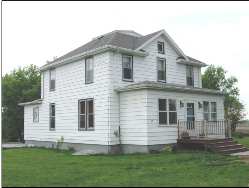
Figure 3–94. View to southeast of residence Building 1 west primary façade and north elevation.
