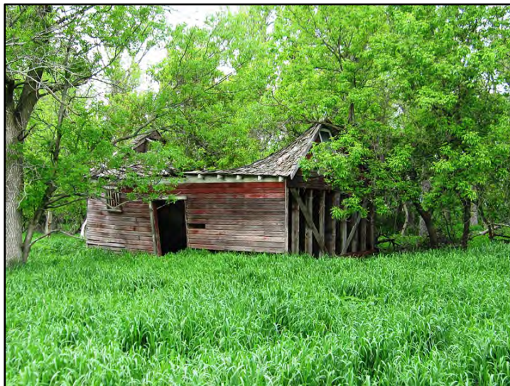
Figure 3–122. View to northwest of Building 7.
