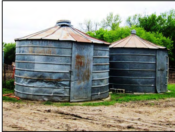
Figure 3–42. View to southwest of grain bins (Building 9) north façades.
