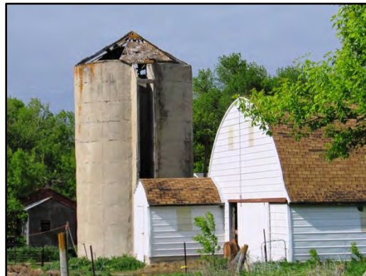
Figure 3–88. View to north of silo and silo chopper house located on northwest side of Quonset barn.
