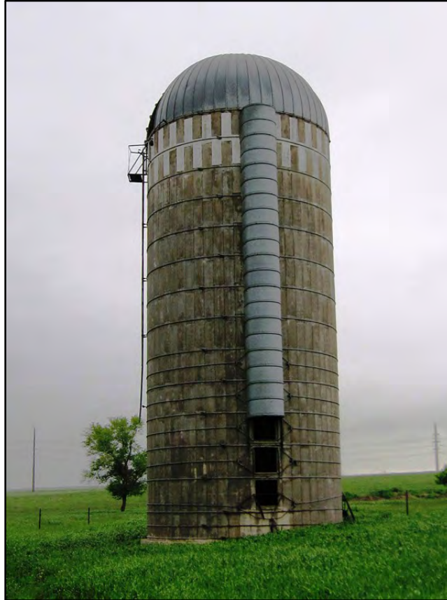
Figure 3–22. View to north of Stansky farm concrete stave silo south façade.
