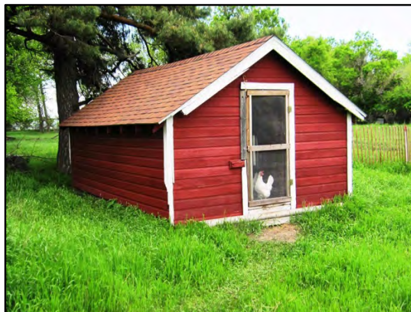
Figure 3–49. View to northeast of chicken coop Building 3 south primary façade and west elevation.
