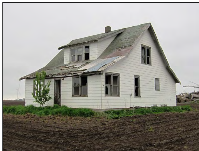
Figure 3–73. View to southeast of Building 1 residence north façade and west elevation.
