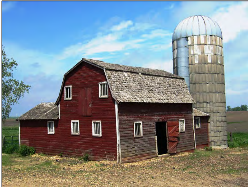
Figure 3–17. View to northeast of Building 3 barn south primary façade and west elevation.
