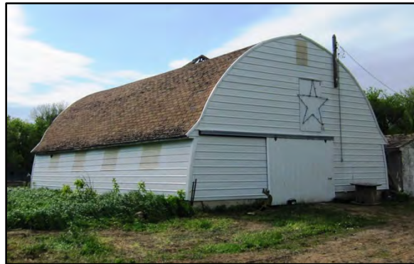
Figure 3–87. View to northwest of Building 4 Quonset barn east primary façade and west elevation.
