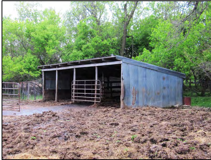
Figure 3–38. View to southwest of Building 5 east primary façade and north elevation.
