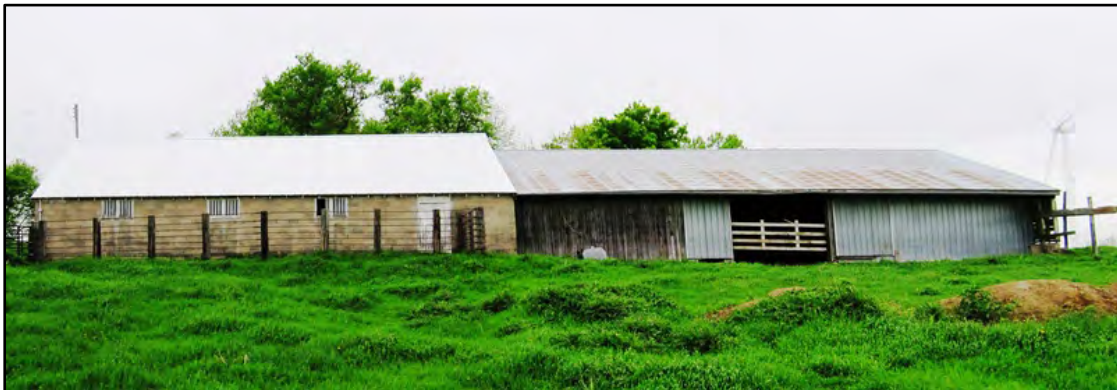
Figure 3–104. View to west of Building 5 (left) and Building 6 (right) east elevations.
