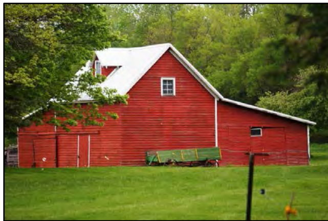
Figure 3–60. View to northeast of granary west primary façade and south elevation.
