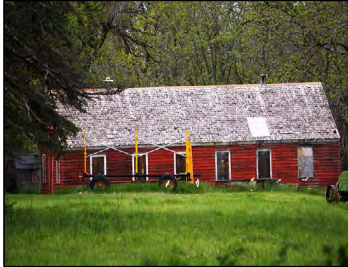
Figure 3–58. View to north of Building 5 south elevation.
