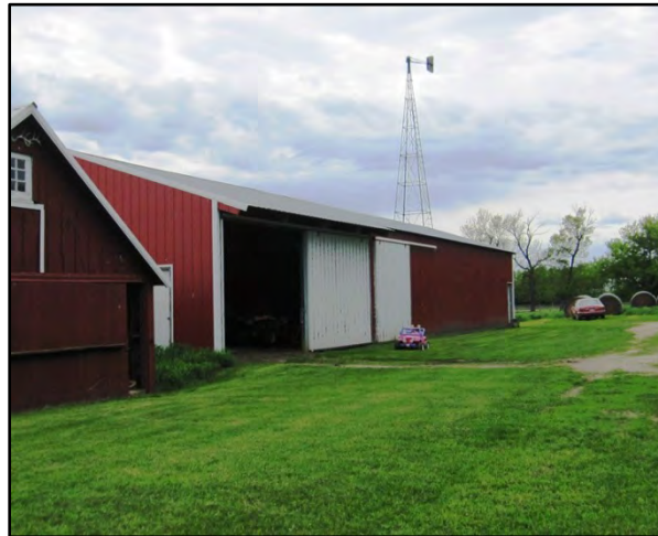
Figure 3–53. View to southwest of Building 8.
