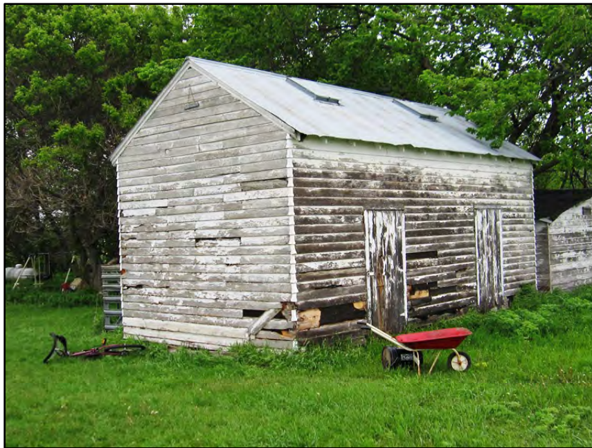
Figure 3–114. View to northeast of Building 4 south primary façade and west elevation.
