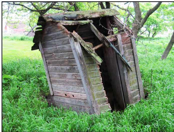
Figure 3–95. View to northeast of privy Building 2 south primary façade and west elevation.
