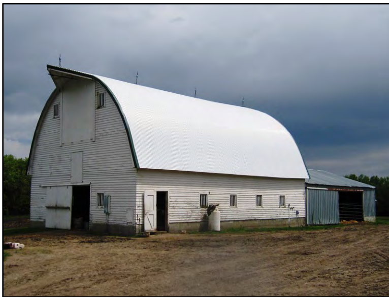
Figure 2–12. This Gothic arch roof wood-clad dairy barn is situated at site BK00001244 in the project area. The Moen family farmed at this site for nearly 70 years. Note the fixed sash wood windows with four vertical mullions, a common window type seen in the study area historic age buildings.
