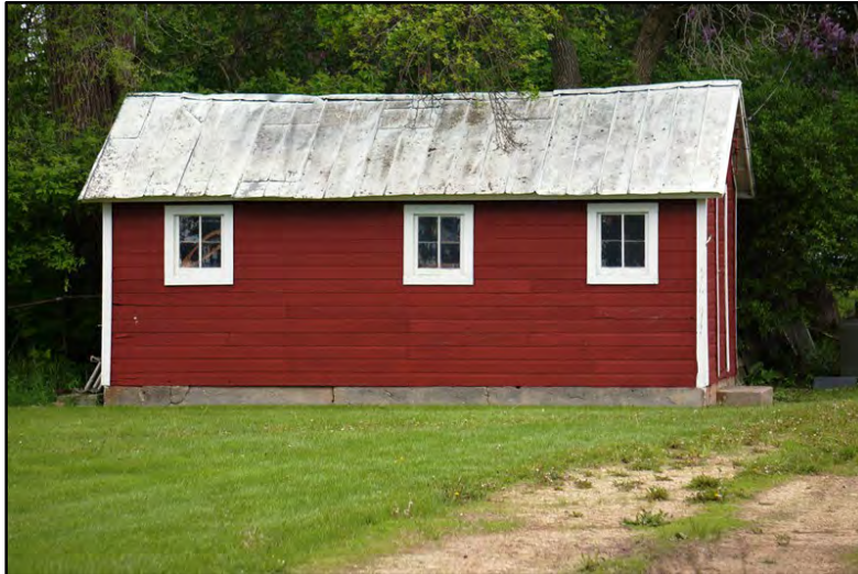
Figure 3–56. View to east of Building 3 west elevation.
