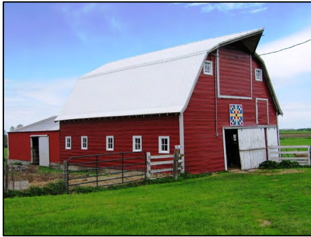
Figure 3–66. View to northeast of barn Building 5 south primary façade and west elevation.
