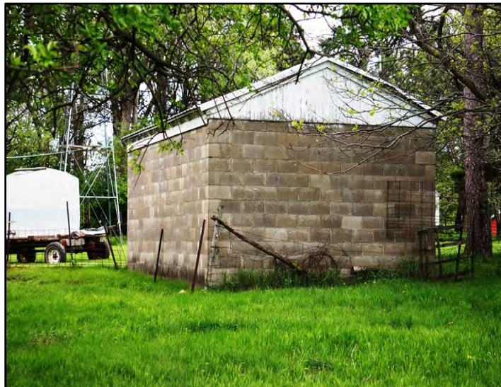
Figure 3–54. View to southeast of Pump house Building 1.
