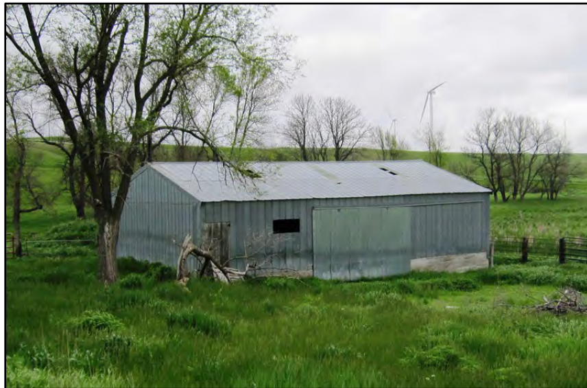
Figure 3–5. View to northeast of Building 2 modern age feed shed south primary façade and west elevation.
