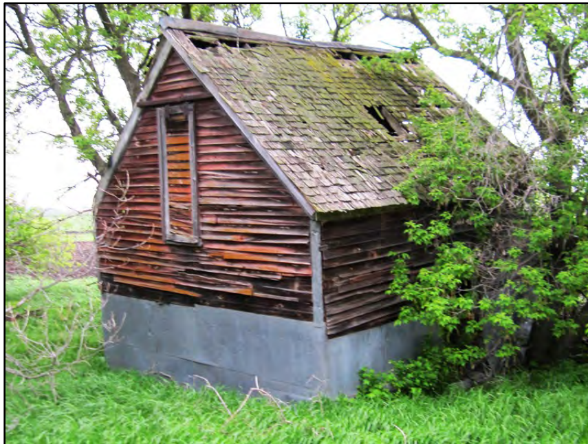
Figure 3–111. View to southeast of granary Building 2 south and west elevations.
