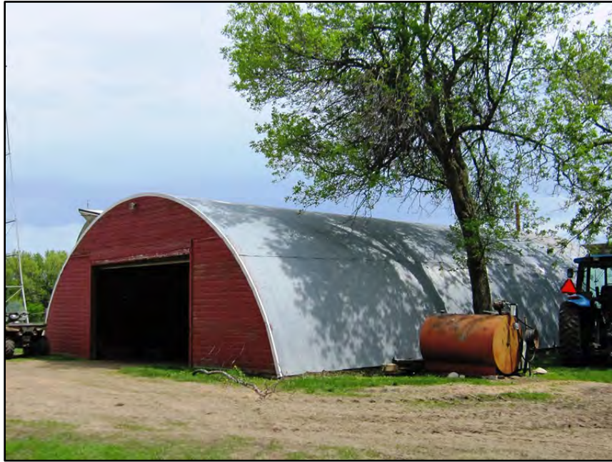
Figure 3–40. View to southeast of Building 7 north façade and west elevation.
