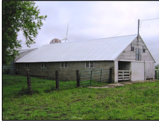
Figure 3–103. View to northeast of Building 5 south primary façade and west elevation.
