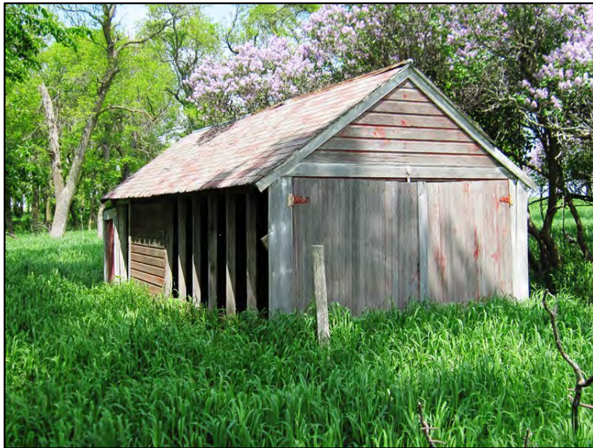
Figure 3–118. View to north of garage Building 2 south primary façade and west elevation.
