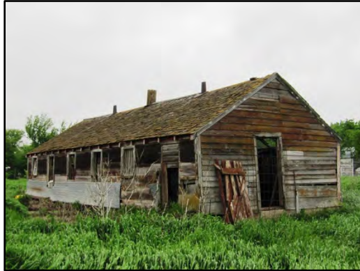
Figure 3–115. View to northwest of Building 5 south primary façade and east elevation.
