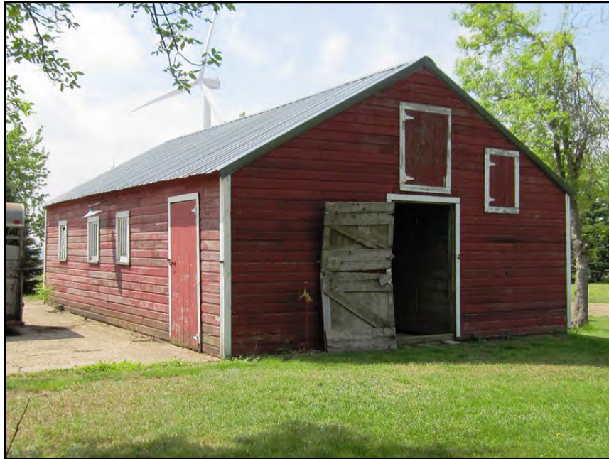
Figure 3–18. View to northwest of Building 4 stable east primary façade and south elevation.
