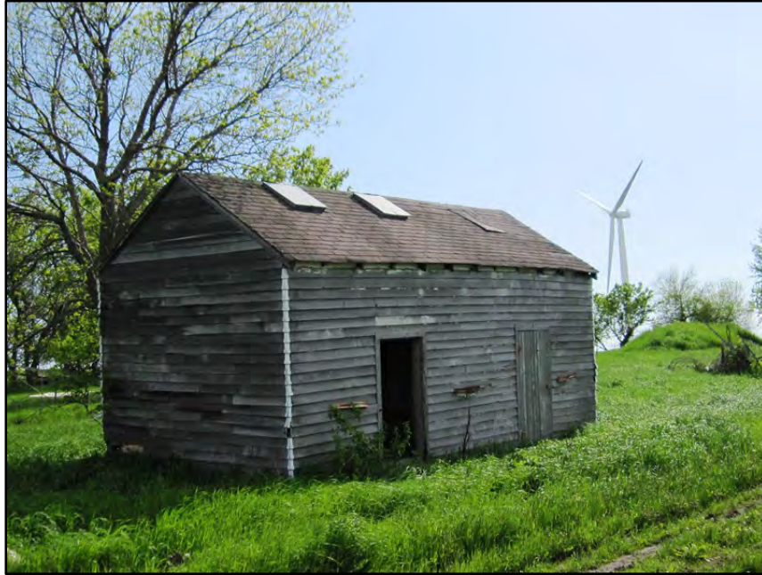
Figure 3–93. View to southwest of Building 9 north primary façade and east elevation.
