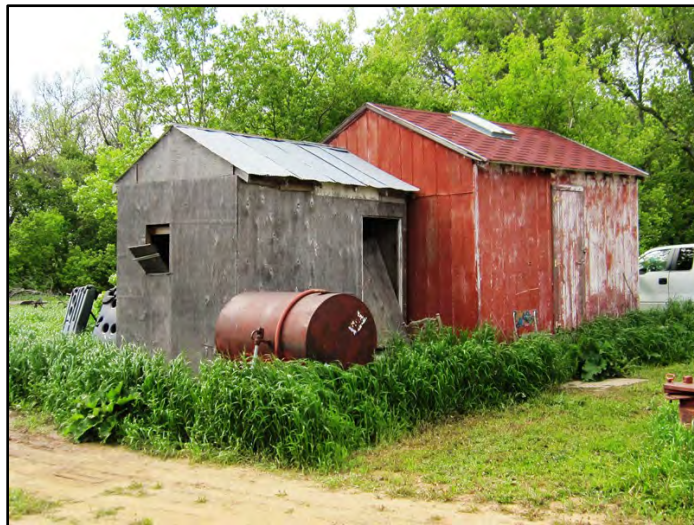
Figure 3–86. View to northwest of Building 3 east facades and south elevations.
