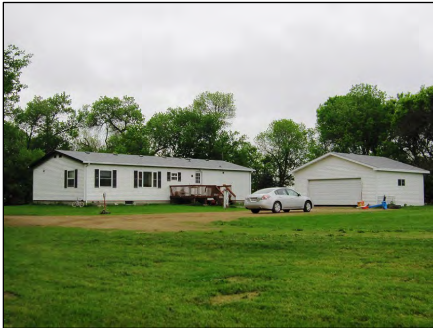
Figure 3–112. View to northeast of Building 1 residence and Building 2 garage.
