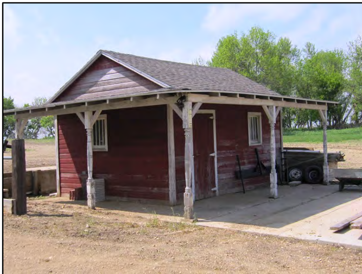
Figure 3–16. View to northwest of Building 2 storage building east primary façade and south elevation.
