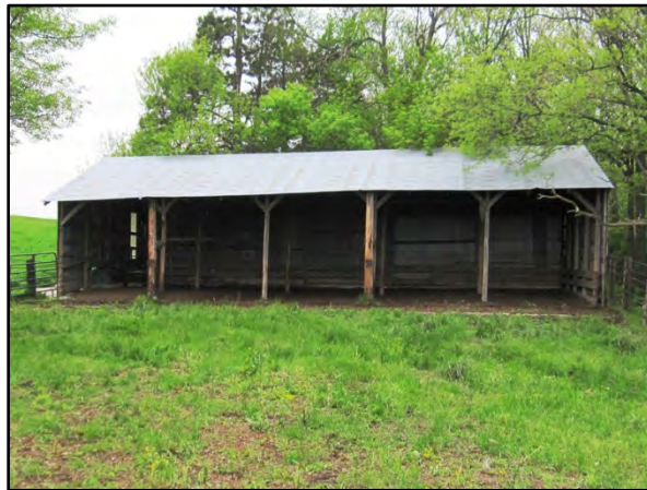
Figure 3–102. View to west of feed shed Building 4 east primary façade.
