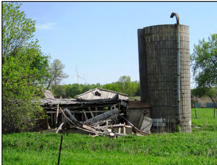
Figure 3–77. View to southwest of Building 4 silo and collapsed Building 5.
