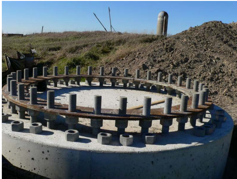
Figure 4. Pier Foundation
