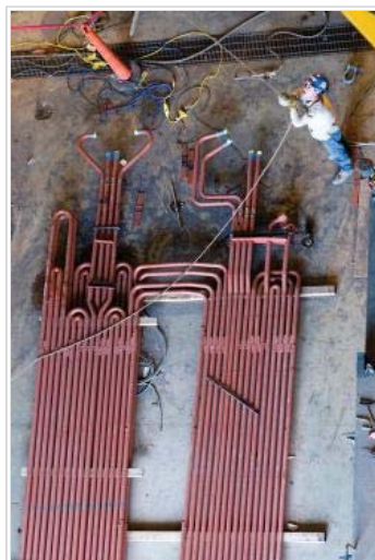
A worker holds a rope tied to a set of pipes being raised into the boiler at the WyGen III power plant. The plant is about 60 percent complete. - News-Record photo by Nathan Payne
