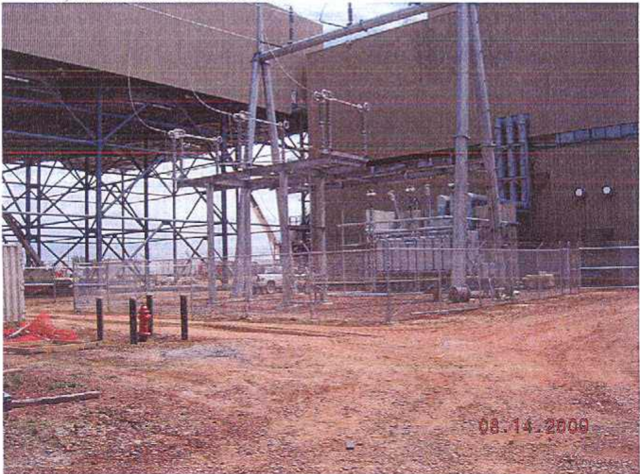
Transformer Yard Progress
