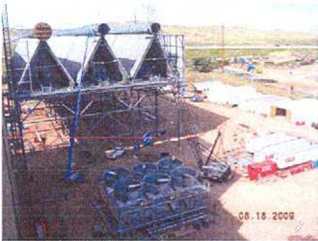
ACW/ACC Erection Progress
