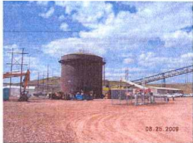
Service Water Storage Tank
