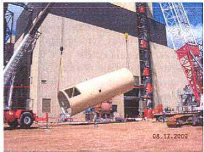
PAC Silo Installation
