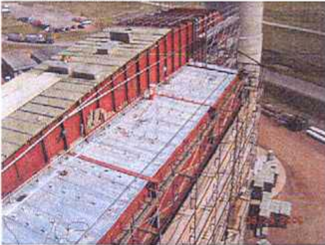
Baghouse Insulation and Lagging
