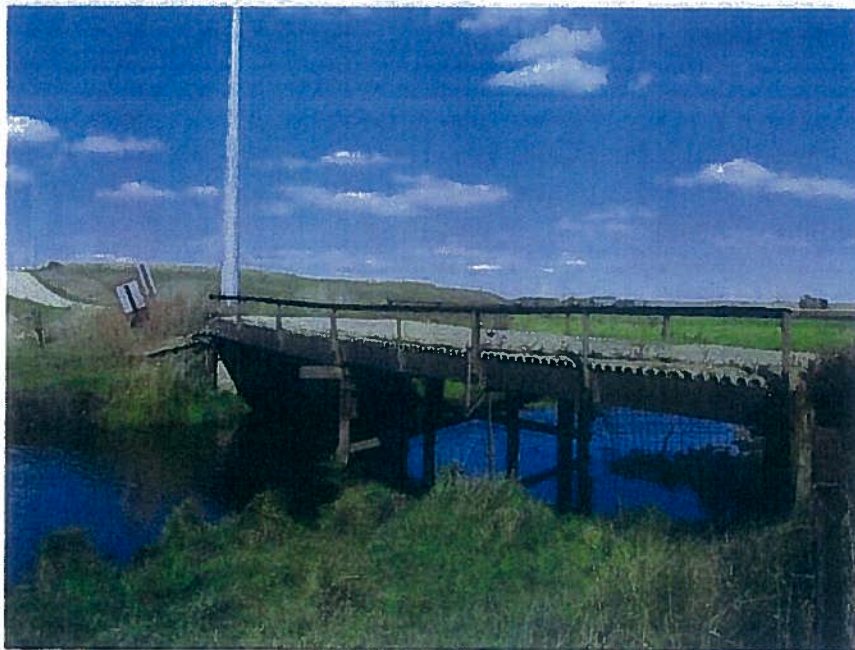
Bridge on 484th Ave south of 207th St
