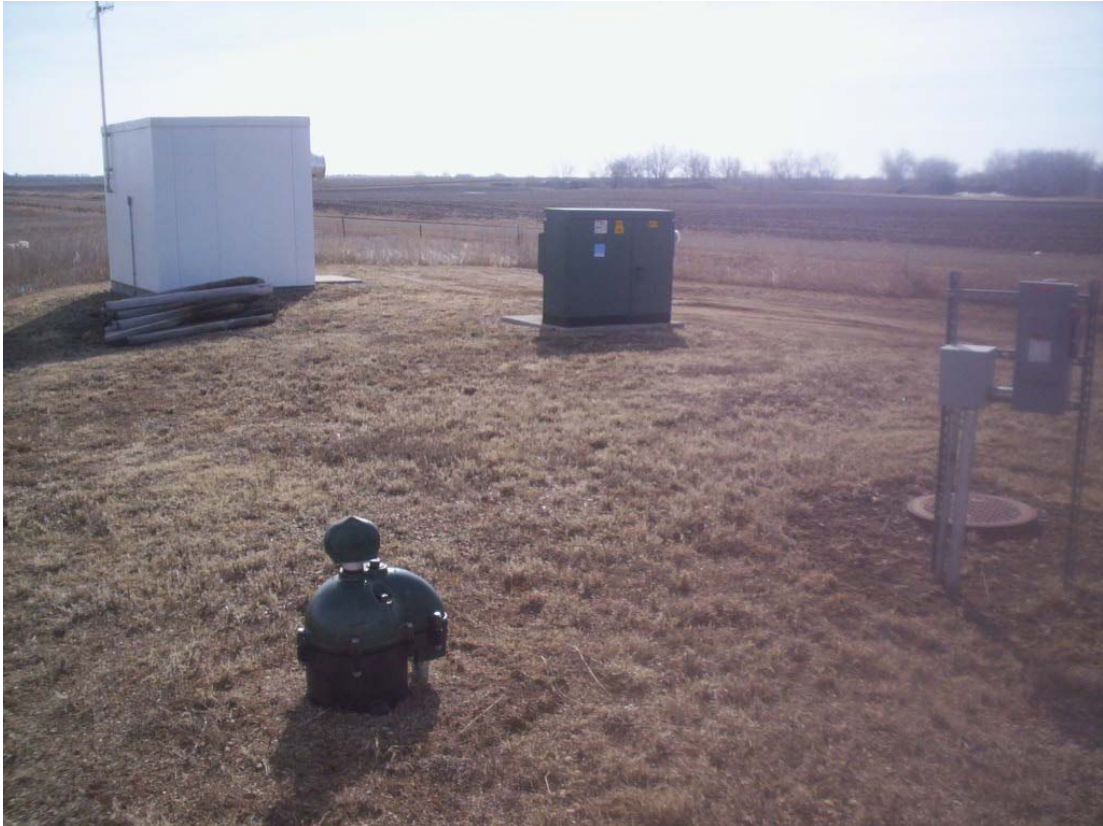
Exhibit 3.4-6: Photo of Typical Well Site
