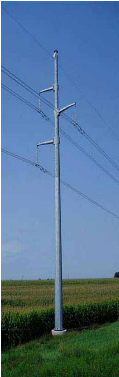
Figure 6: 115 kV Single-Circuit Davit Arm Structure
