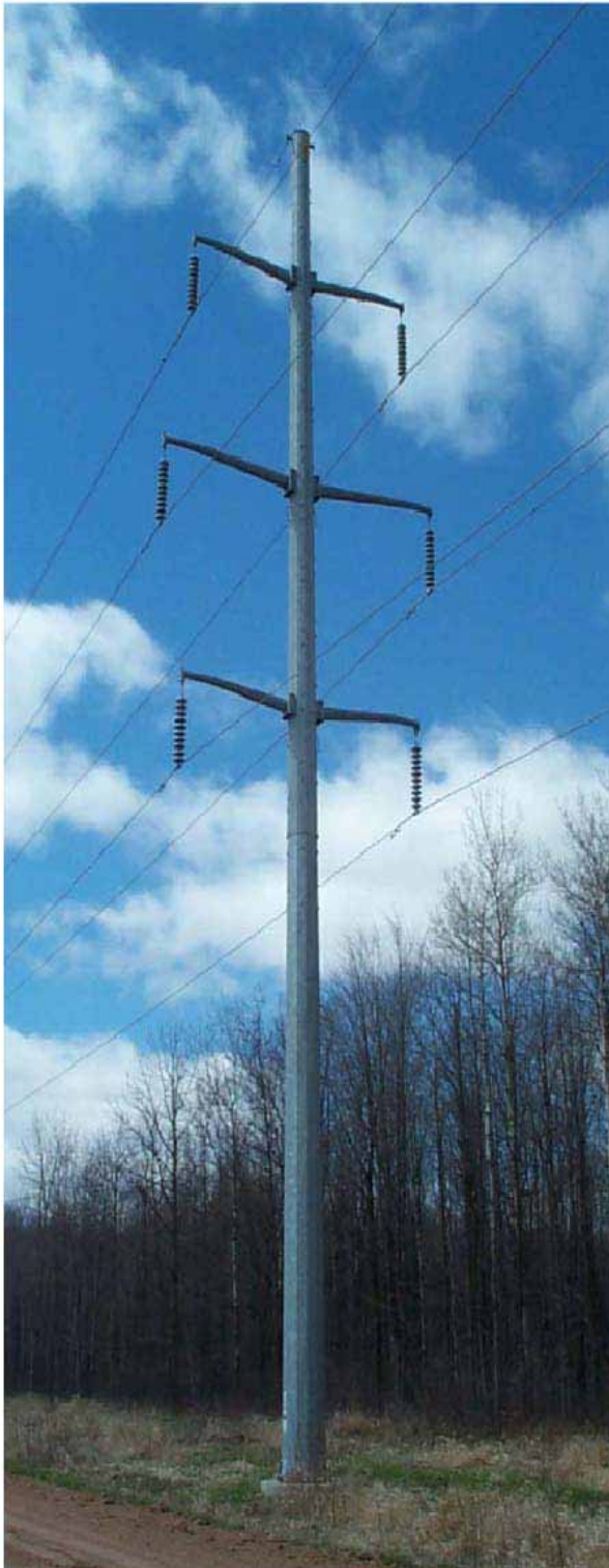
Figure 7: 115 kV/115 kV Steel Double-Circuit Davit Arm Structure
