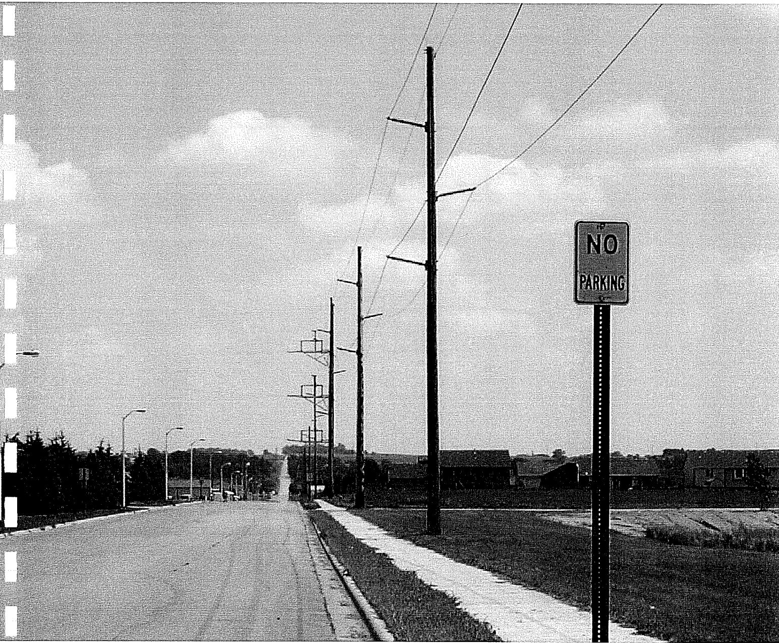
Side Mount 115 kV Insulators
