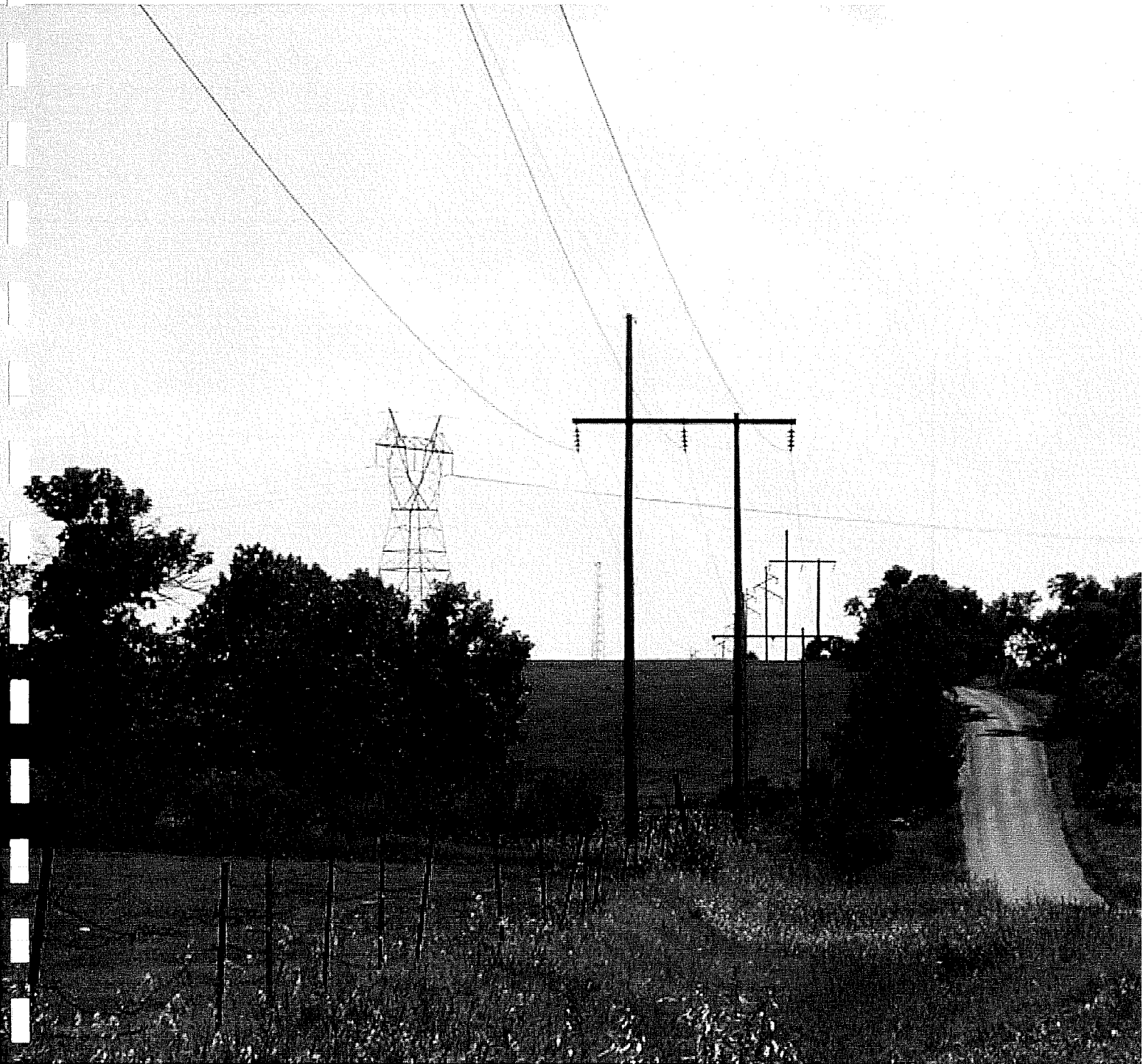
69 kV Two Pole Line Structure with Suspension Insulators
