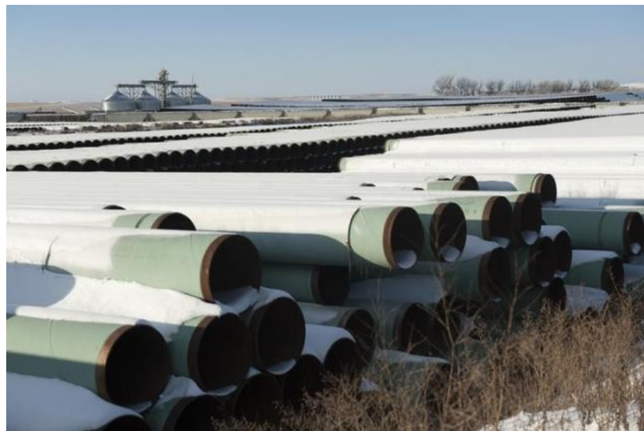
A depot used to store pipes for TransCanada Corp's planned Keystone XL oil pipeline is seen in Gascoyne, North Dakota November 14, 2014. REUTERS/ANDREW CULLEN
