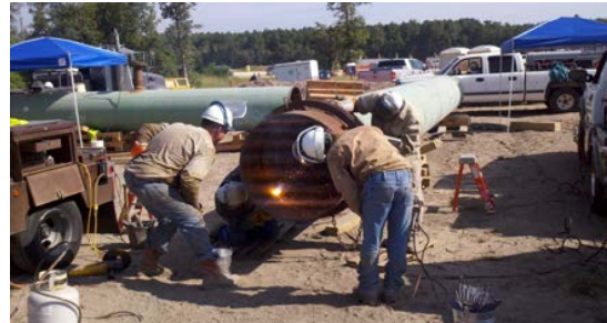
Figure 19: Welder Qualification Test
