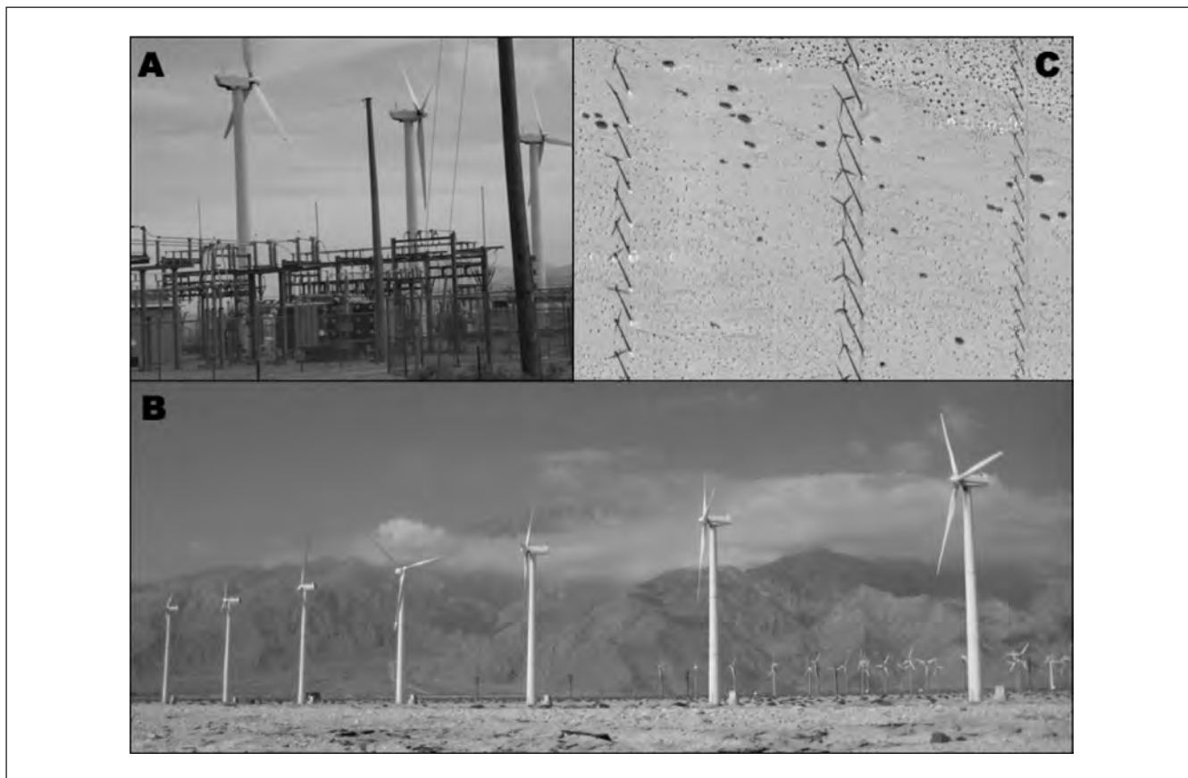
Figure 5. Wind farm in Palm Springs, California, showing (A) location of ground voltage readings; (B), view of wind turbines from the ground; and (C) view of wind turbines from the air Note. Photograph A from Dr. Sam Milham. Photographs B and C from Google maps.
