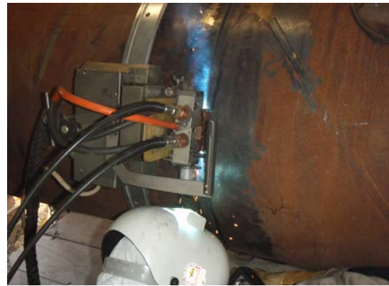
Figure 21: Automatic Welding Set up
