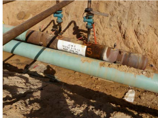
Figure 28: Hydrotest in Progress
