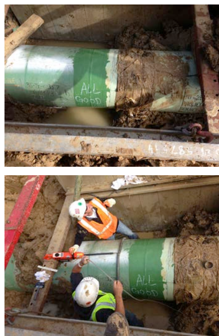
Figure 25 and 26: DCVG dig site (recoated)
