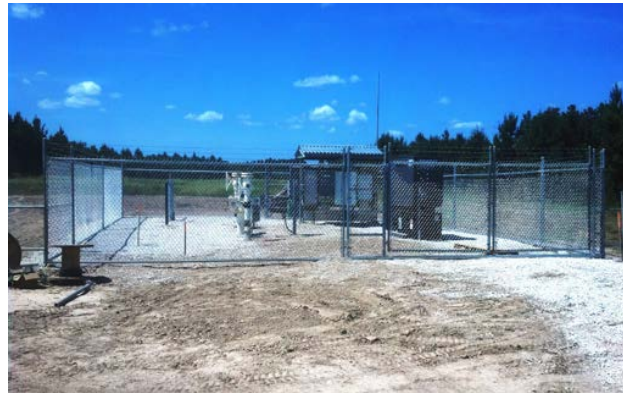
Figure 18: Typical Fencing around Valve site
