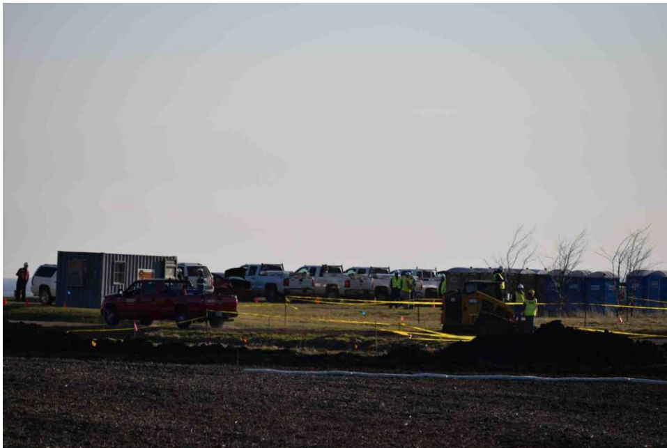
On this visit, 437 th Avenue seemed to be intact with piles of dirt on each side. *Photo 0864.
