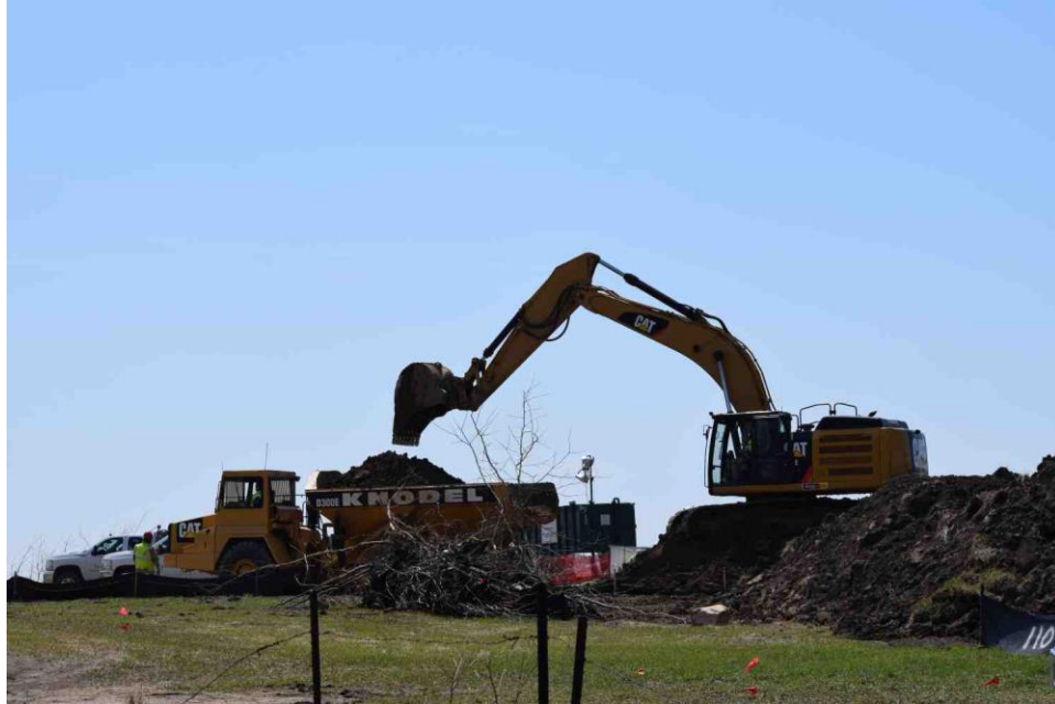
The spill site was at the top of a hill, and it seems any water-soluble contaminants, such as benzene, could have easily washed down the hillside. *Photo 1053.
