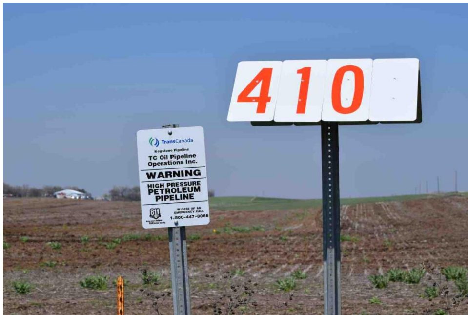
Recent rains caused visible washing across a barren field at the northeast corner of the intersection of Highway 18 and 437 th Avenue. To the south across the Highway, at the top of a hill, was a pile of excavated dirt from the spill site. *Photo 1067.
