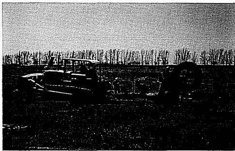
We are building new communication highways with fiber optic cables.
