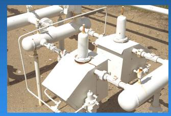
6) Pipe or Components subject to Clogging must have Provisions for Cleaning
