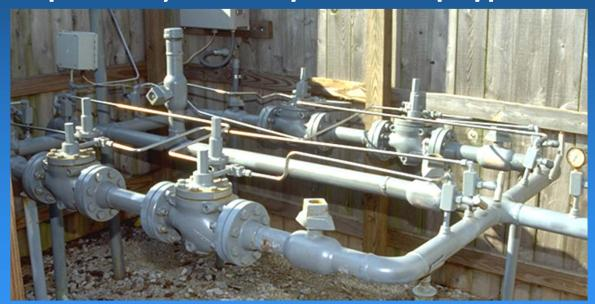
9) Damage to Any One Control Line may not make both the Regulator and Protective Device Inoperative.
