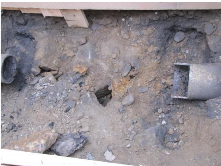
Figure 16: 12-inch water main pipe with circumferential crack bottom view.
