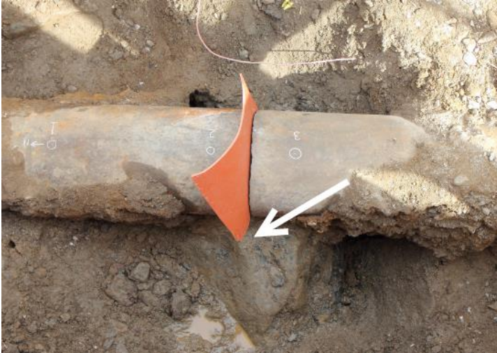
Figure 15: 12-inch water main cracked location directly located on top of rock.
