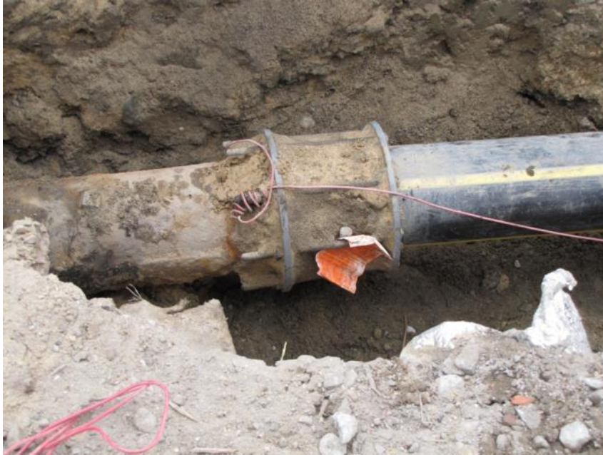
Figure 3: North end of 8-inch HDPE gas main joined to 8-inch cast iron pipe to the left with 8-inch steel mechanical coupling in front of 1644 Park Avenue.
