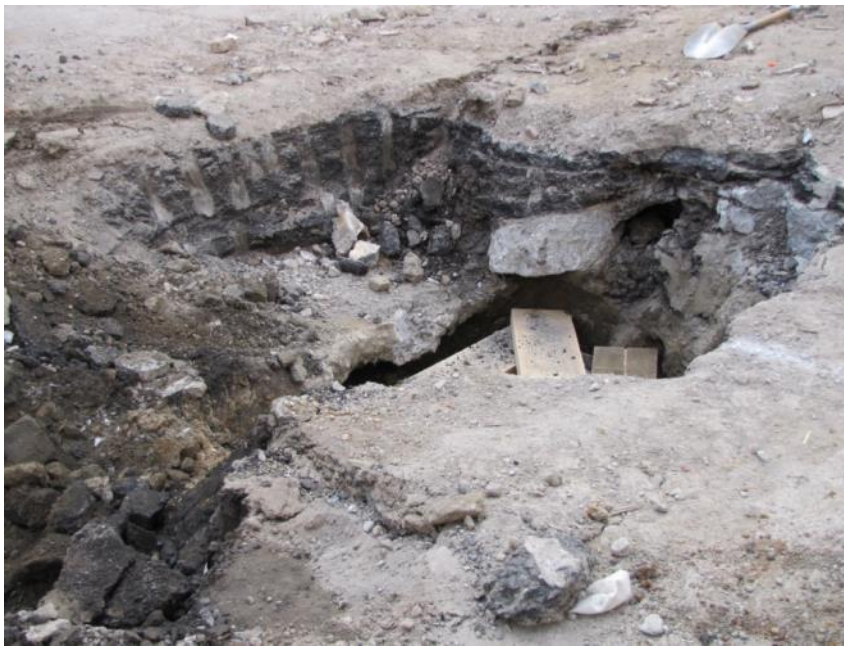
Figure 31: Excavation showed layered roadway and large horizontal void in front of 1644 and 1646 Park Avenue.
