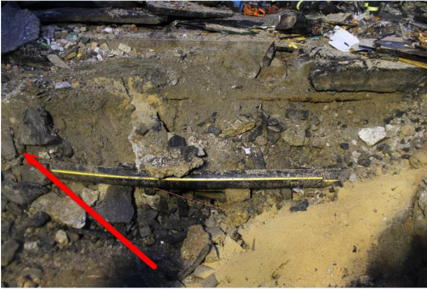
Figure 12: The exposed 8-inch HDPE gas main and top of 2-inch HDPE service saddle tee indicated with a red arrow, in front of 1642 Park Avenue. Source: NYPSC.
