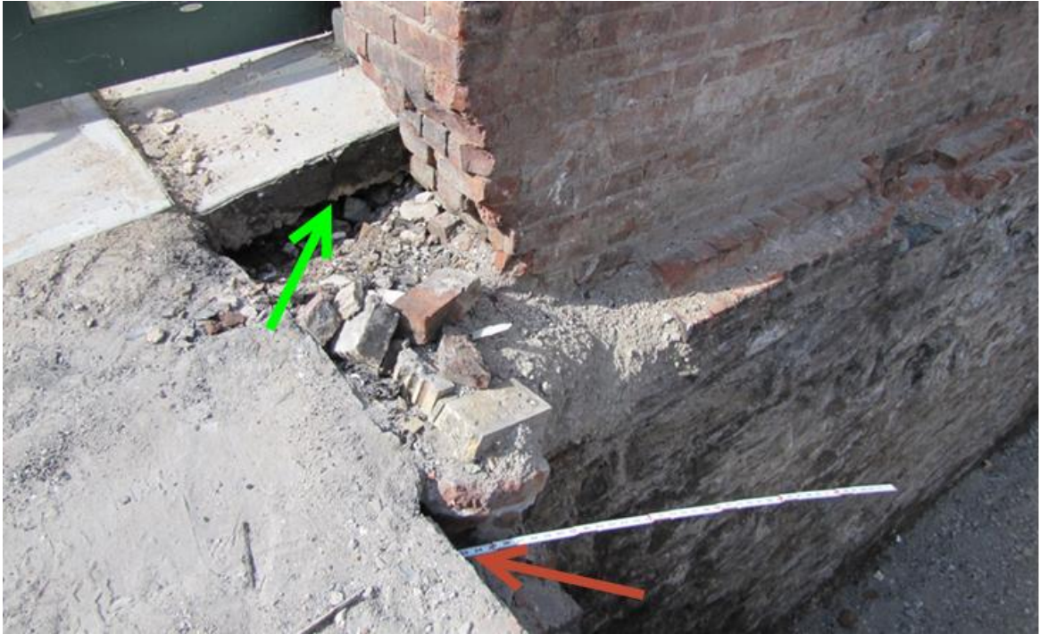
Figure 32: Underneath slab openings at 1642 and 1644 Park Avenue.
