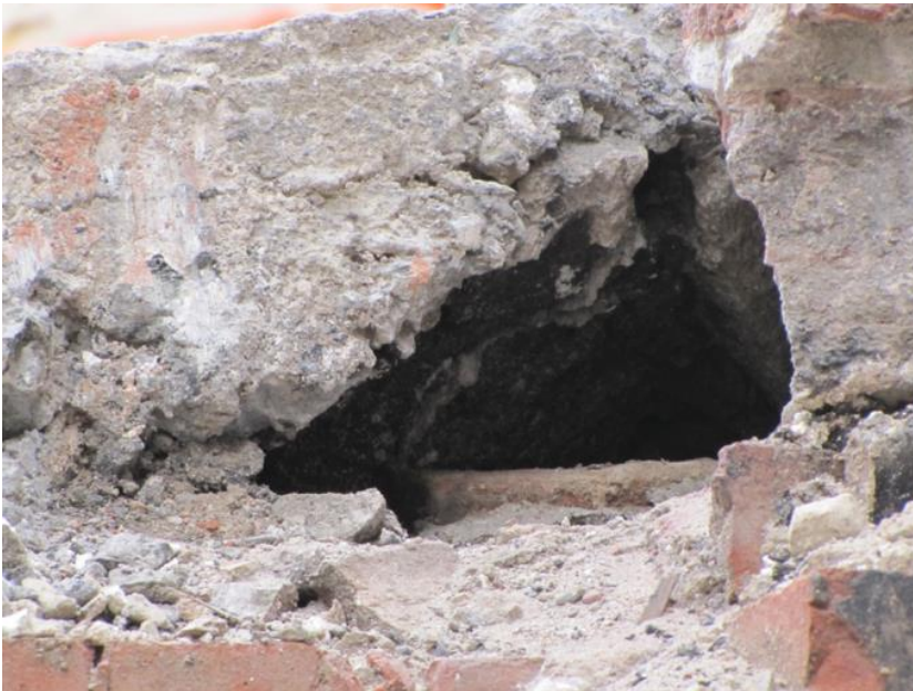
Figure 33: Hole at 1644 Park Avenue frontage under sidewalk slab.
