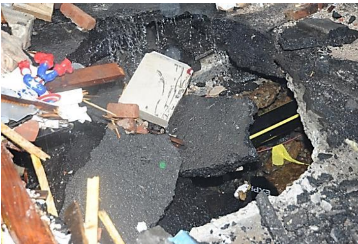
Figure 11: Sink-hole at 12-inch cast iron water main break location showing 8-inch HDPE gas main. Source: FDNY
