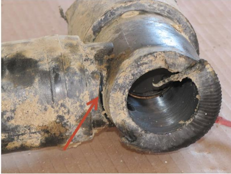
Figure 27: Underside of the saddle tee showing the tee to gas main fusion surface and crack in the service line connection port (red arrow).
