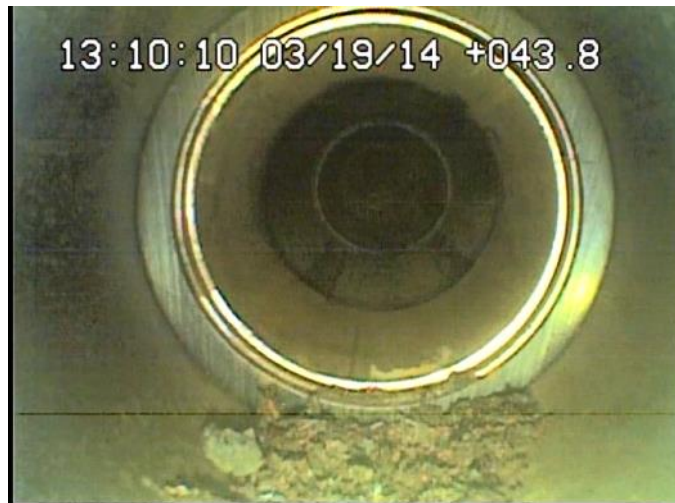
Figure 20: Internal camera inspection of 8-inch gas main pipe shows transition from cast iron to HDPE. Source: Con Edison
