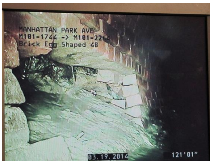
Figure 6: Damaged east side of sewer main wall (12 inches by 40 inches) in front of 1644 and 1646 Park Avenue. Source: NYCDEP
