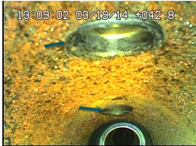
Figure 19: Internal camera inspection of 8-inch gas main pipe shows two 2-inch plugs at about 43 feet and 44 feet. Source: Con Edison
