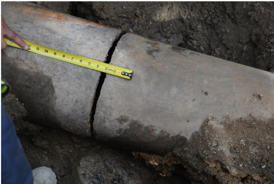
Figure 14: 12-inch cast iron water main pipe with circumferential crack top view. Source: NYCDEP
