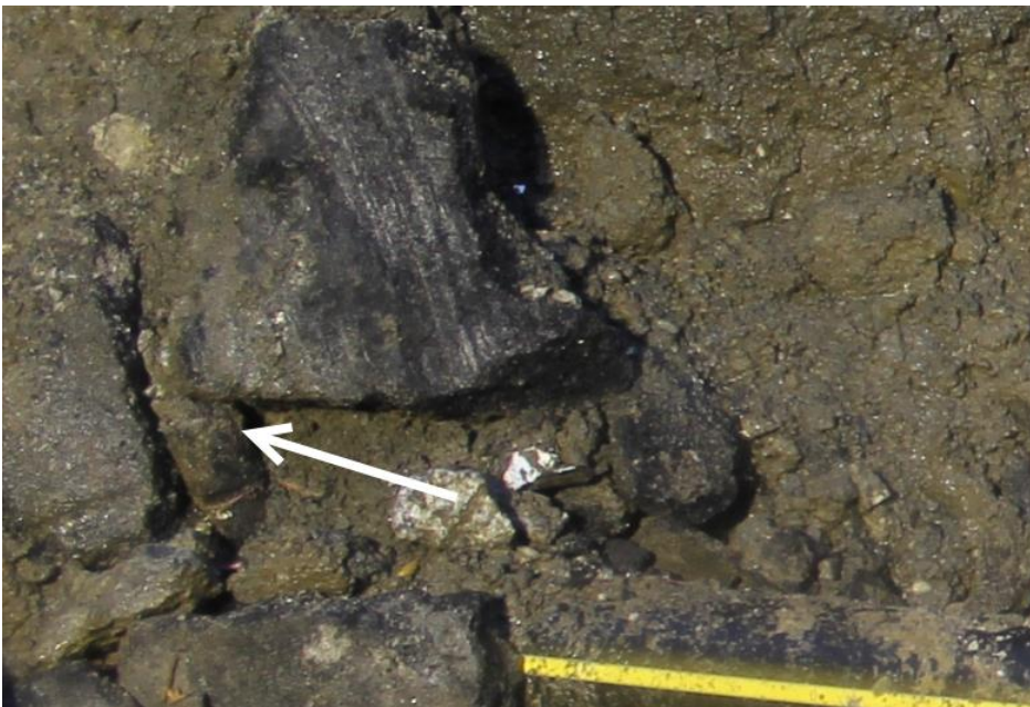
Figure 13: Close view of exposed 8-inch HDPE main and top of 2-inch HDPE service saddle tee indicated with a white arrow, in front of 1642 Park Avenue. Source: NYPSC.
