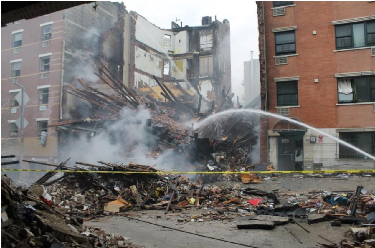
Figure 1. Explosion damage to 1644 and 1646 Park Avenue.
