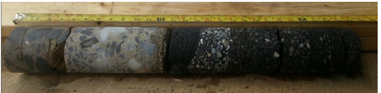
Figure 30: Core #6 road pavement sample from front of 1646 Park Avenue near incident properties service tees. Source: Con Edison.
