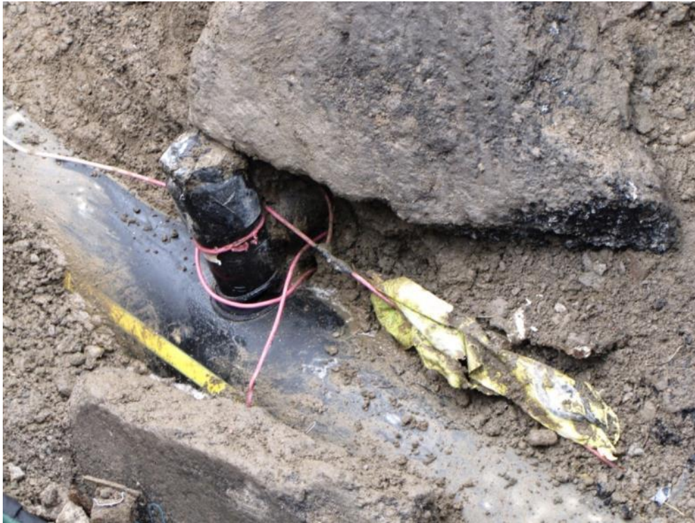
Figure 23: Separated gas service saddle tee at 1642 Park Avenue.
