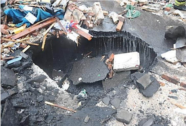
Figure 10: Sink-hole at the location of the 12-inch cast iron water main break. Source: FDNY
