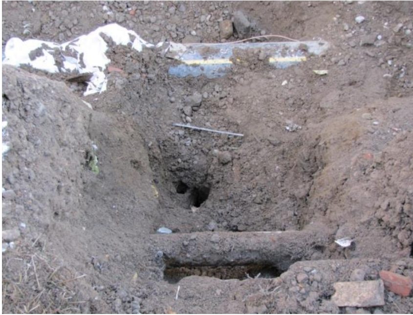
Figure 26: Porous soil and large holes at 1642 Park Avenue near the gas main.
