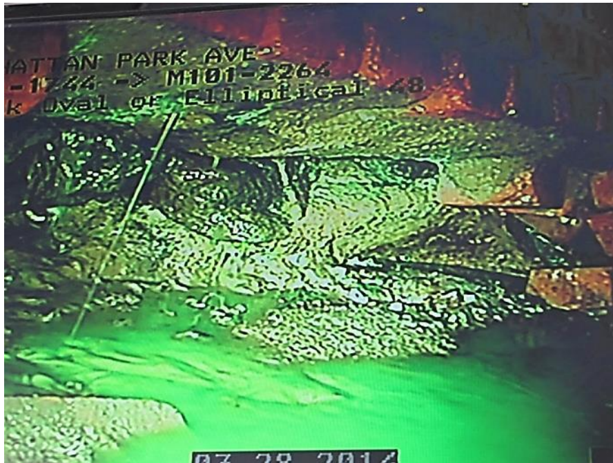
Figure 18: Florescent Green dyed water solution entering the sewer main at (hole-B) the damaged east sidewall. Source: NYCDEP
