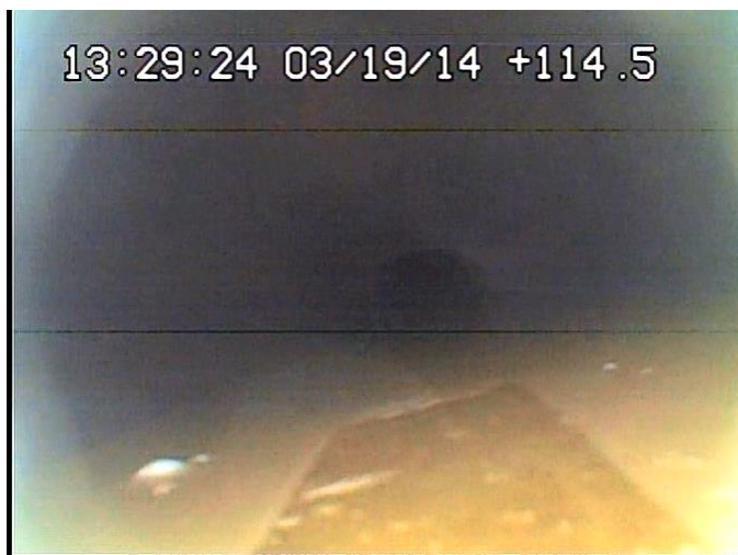
Figure 22: 8-inch gas main pipe with pool of water in the main PE pipe. Source: Con Edison
