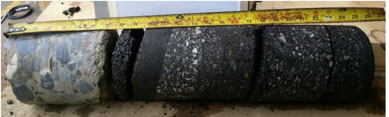
Figure 29: Core #4 road pavement sample from front of 1646 Park Avenue near incident properties service tees. Source: Con Edison.
