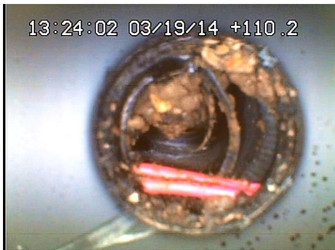
Figure 21: 8-inch HDPE gas main disconnected 2-inch service tee on the main HDPE and red tracer wire. Source: Con Edison
