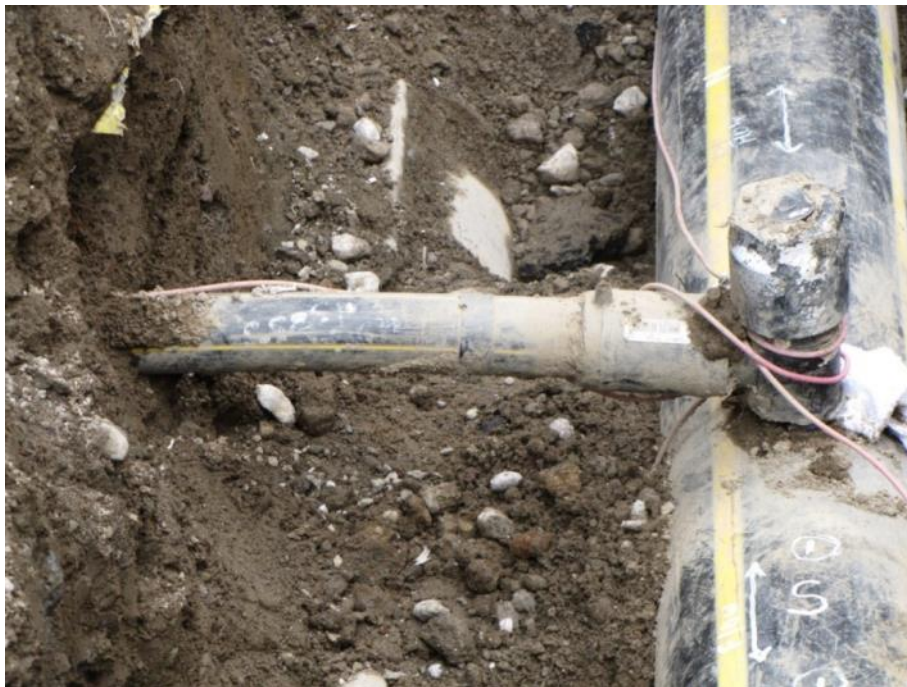
Figure 24: 2-inch separated HDPE service line at saddle tee.
