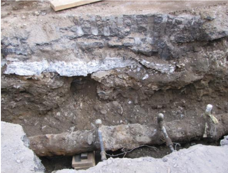
Figure 28: Service tees to 1646 and 1644 Park Avenue below about 12 inches of concrete road underlay with about 18 inches thick asphalt paving.
