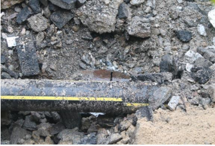
Figure 9: The exposed 8-inch HDPE gas main and 12-inch cast iron water main cracked location.
