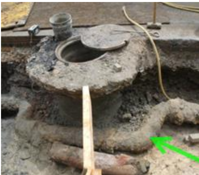
Figure 8: 8-inch cast iron gas main of Con Edison by-passed at upstream manhole of sewer main on Park Avenue, as indicated with green arrow. Source: NYPSC
