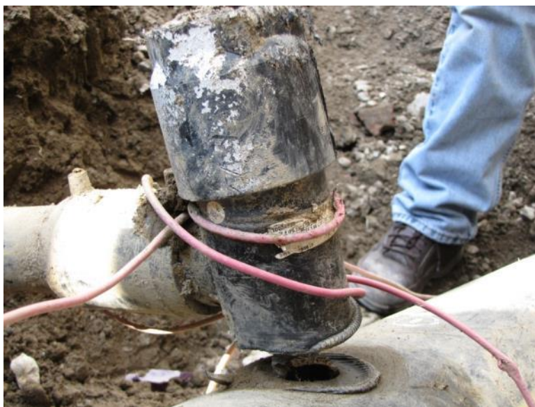
Figure 25: Separated 2-inch saddle tee from the HDPE main.
