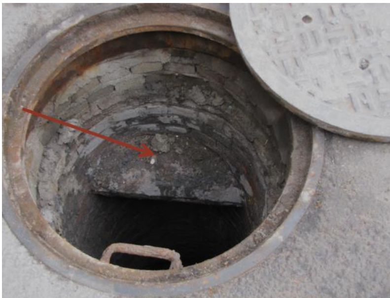
Figure 7: 8-inch cast iron pipe that travel through upstream manhole sewer main at 1652 Park Avenue, as indicated with red arrow at about 1.5 feet below manhole lid and roadway grade.
