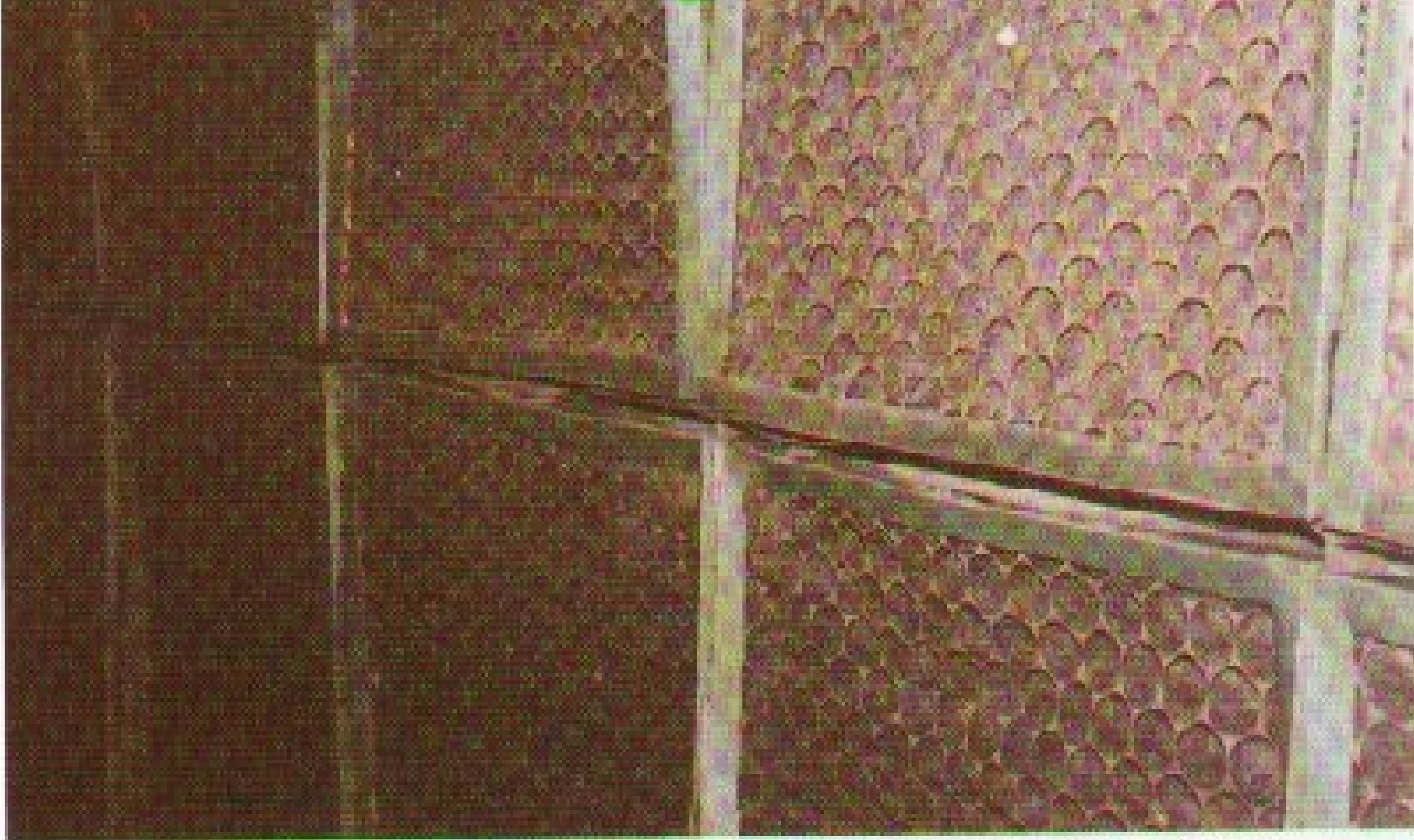
An example of low quality, poorly maintained and improperly fitted filters
